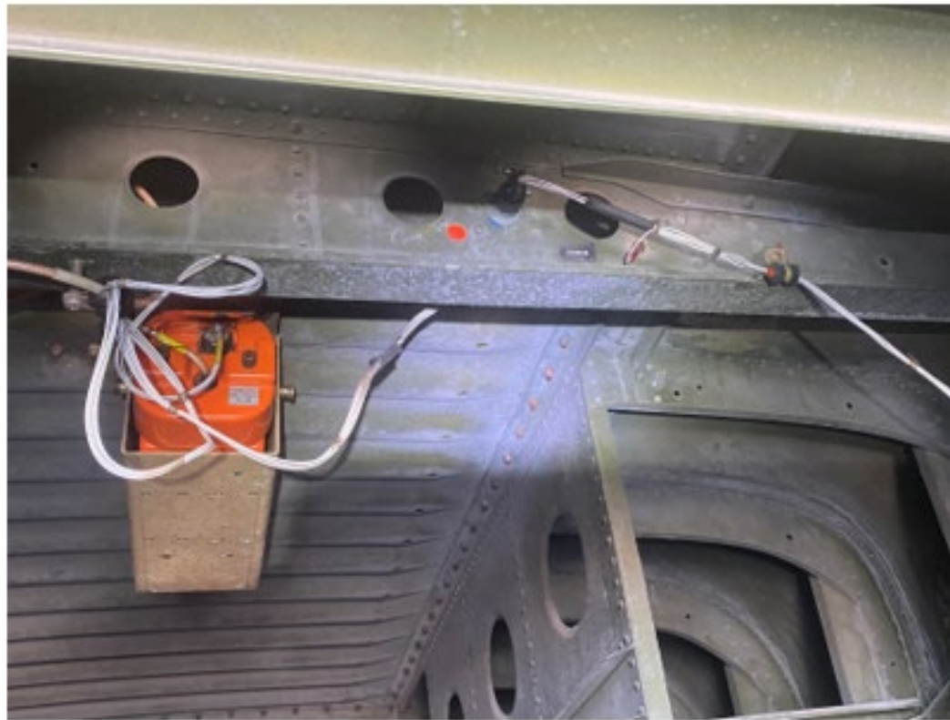
Figure 19 - J310Q Grounding Terminal Corrosion (Discrepancy #16)
