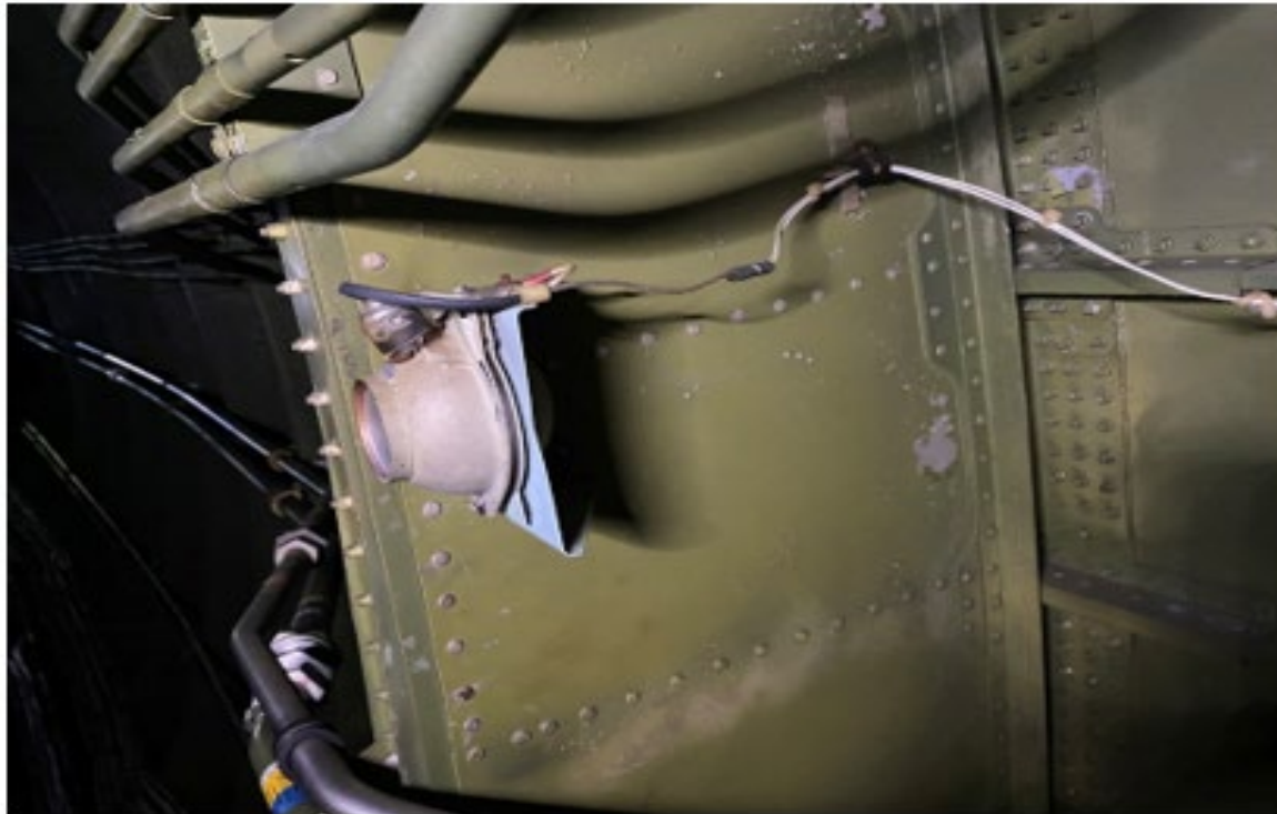
Figure 46 - Wire Insulation Break Down & Loose Screw (FOD) (Discrepancy #43)
