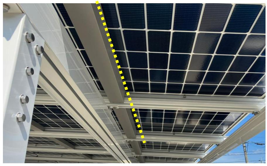
Fix the wiring cover by overlapping it slightly with the vertical rail and screwing
