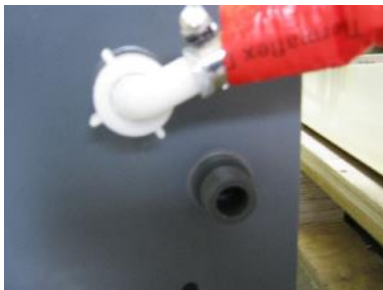
connect the hose to connection from the chiller for „chiller out“
