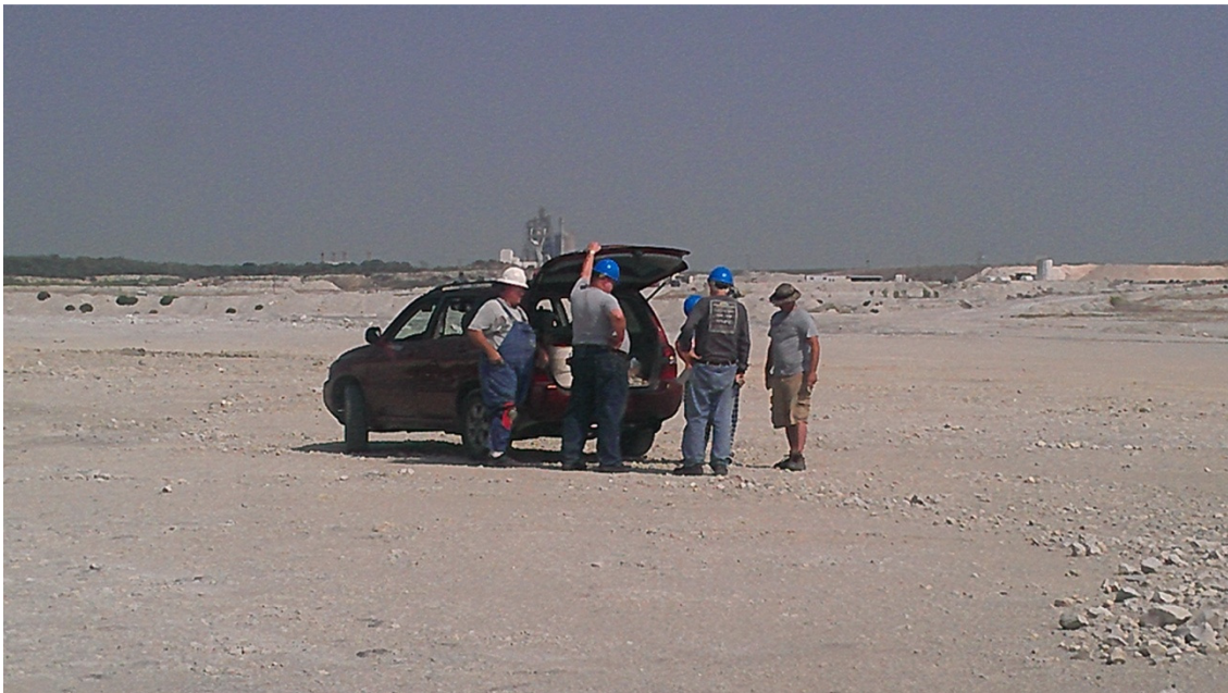
Preparing to dig in Midlothian
