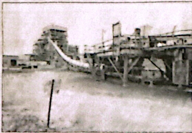
The Gainesville Renewable Energy Center. FILE
