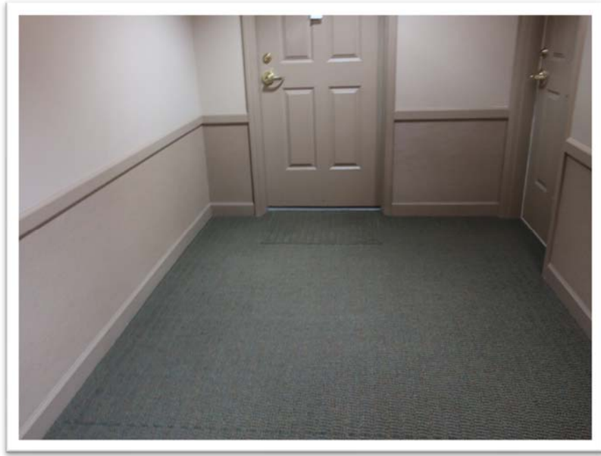
Photograph 9: Typical view of common hallway finishes
