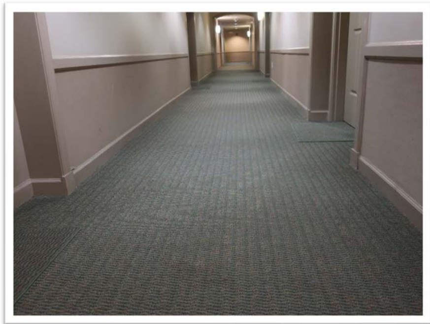
Photograph 12: Typical view of common hallway finishes
