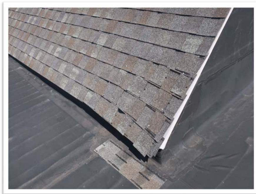
Photograph 4: Typical view of asphalt shingle roof area
