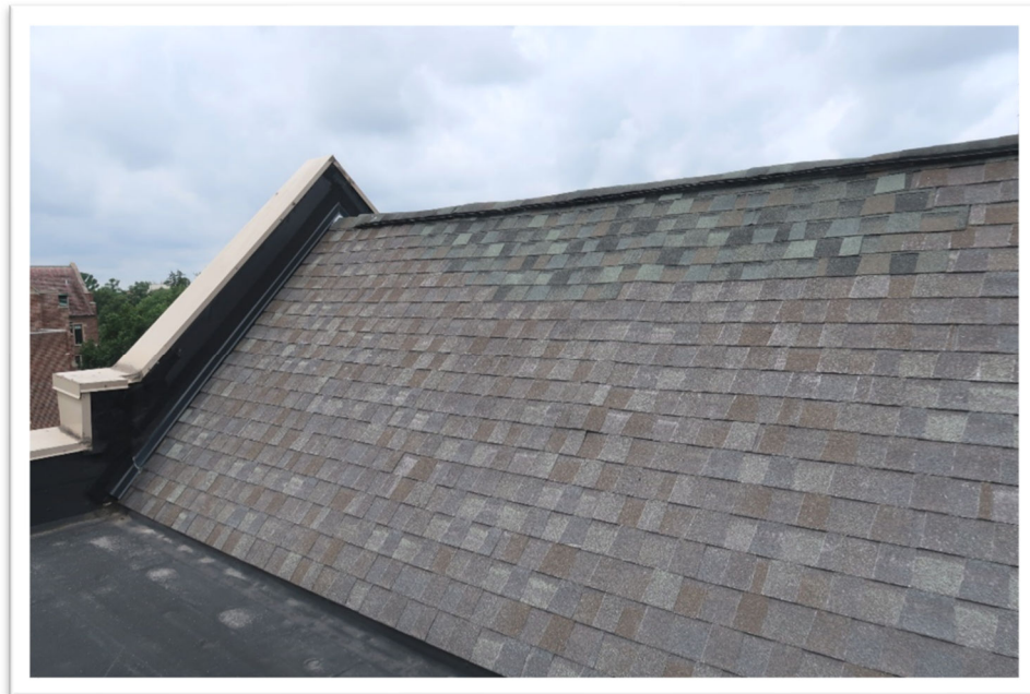
Photograph 4: Typical view of asphalt roof shingles
