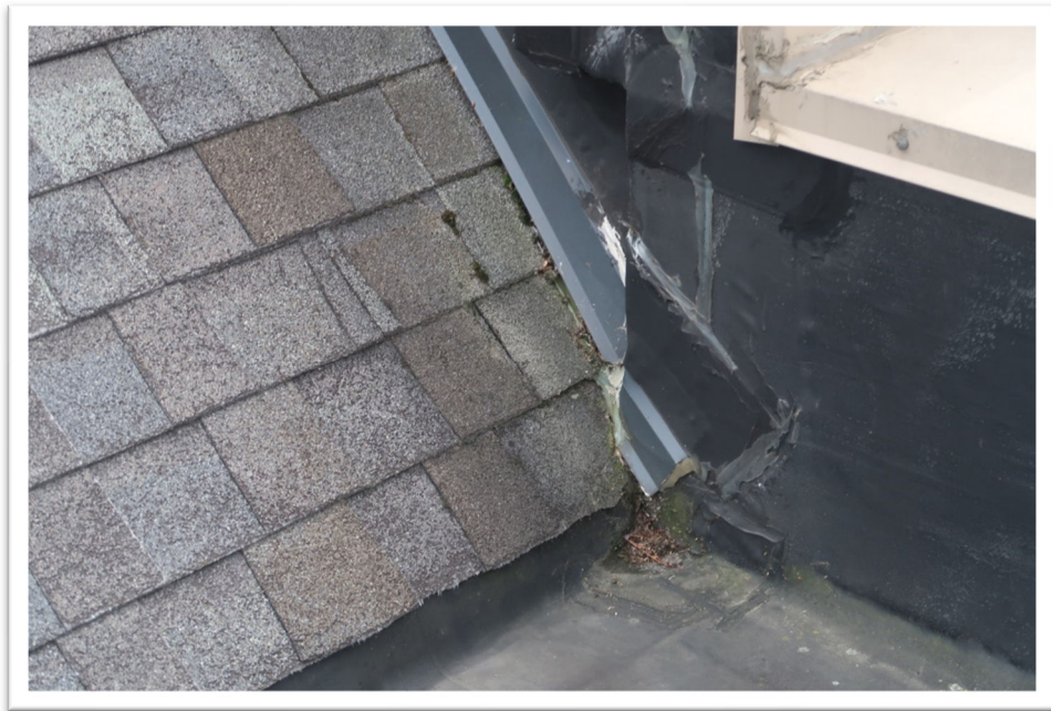
Photograph 7: Typical view of asphalt roof shingles
