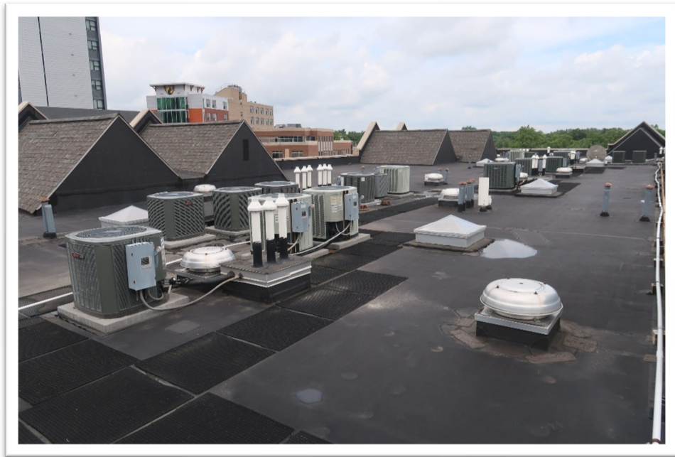
Photograph 9: Typical view of EPDM membrane roof cover
