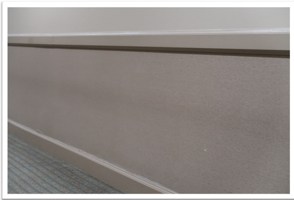
Photograph 17: Typical view of wallpaper
