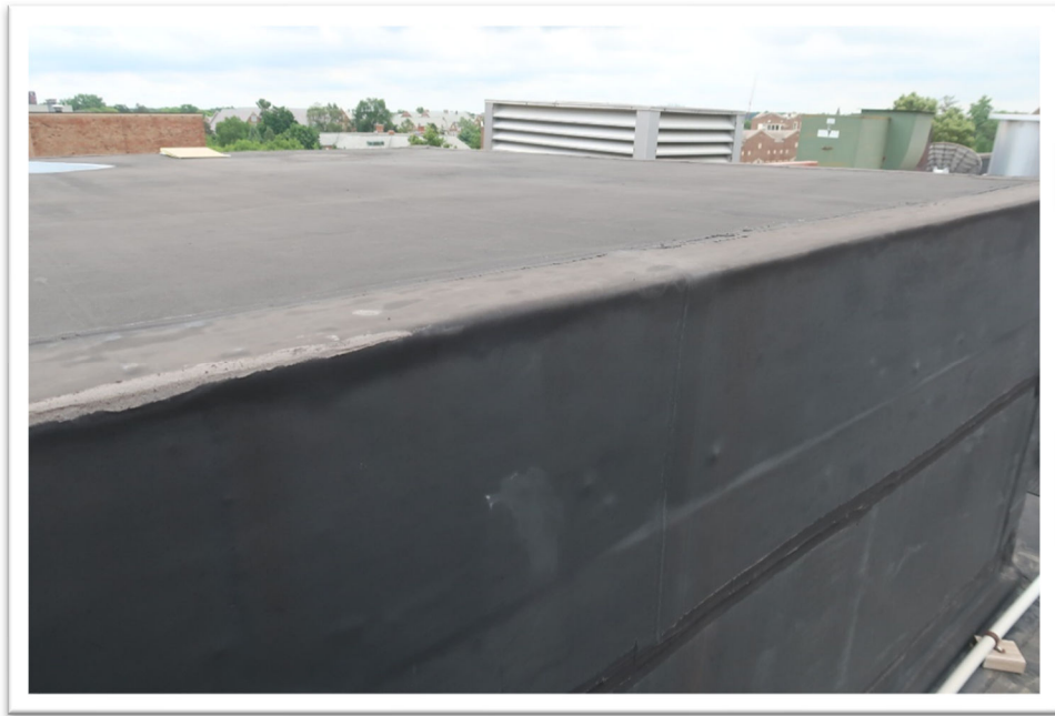
Photograph 11: Typical view of EPDM membrane roof cover
