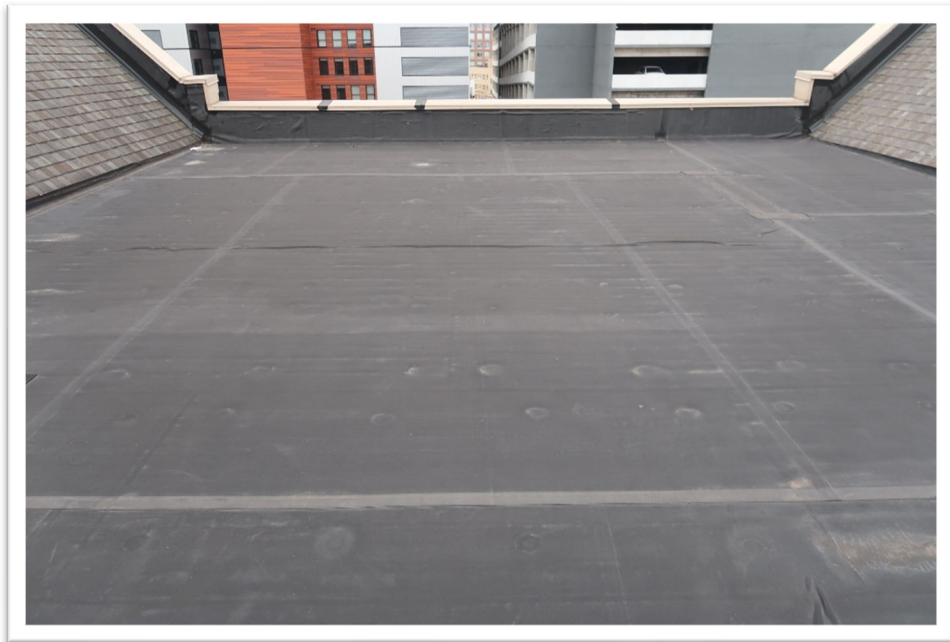
Photograph 10: Typical view of EPDM membrane roof cover
