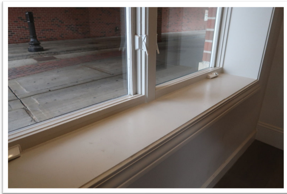
Photograph 13: Typical view of common area window
