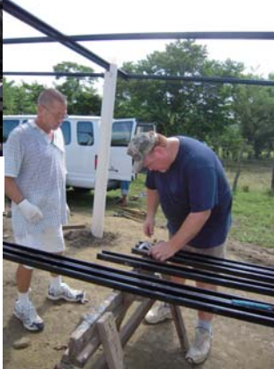
Pastor Mike makes the cuts for metal rafters.
