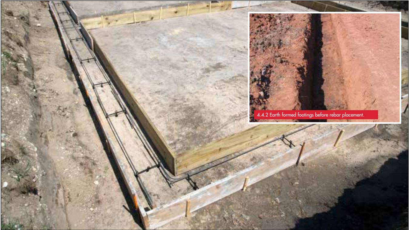
Figure 4.4.1 Footings formed with horizontal rebar in place.
