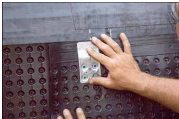
Figure 6.4.5 DMX AG air gap membrane is installed over the peel and stick membrane. This prevents damage from backfill as well as relieves hydrostatic pressure. Do not use screws below grade through the membrane, it will leak.
