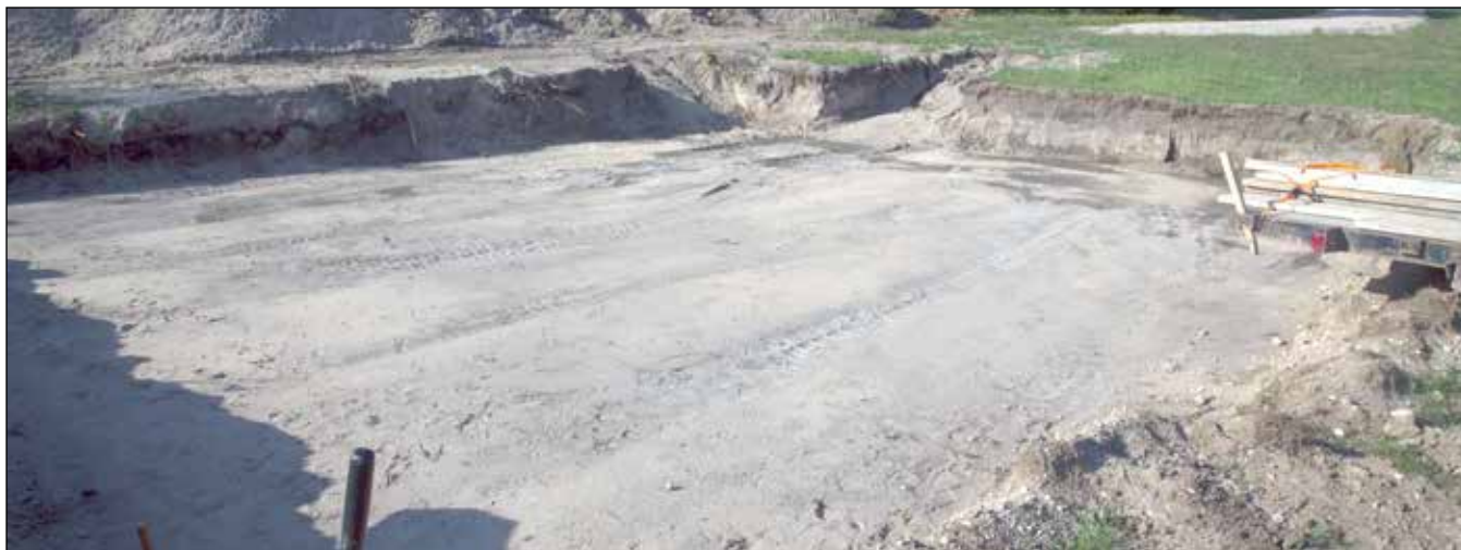
Figure 4.2.1 Typical site excavation staked for square
