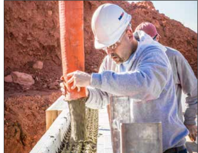
Figure 3.2.2 Pouring concrete into an ICF basement using a pump truck and flat hose.
