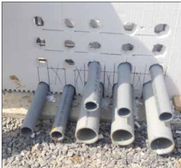
Figure 7.1.1 Complex service penetrations before additional strapping.
