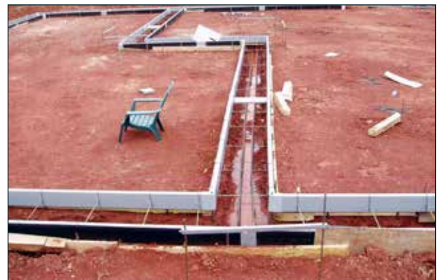
Figure 6.1.4 Form-A-Drain footing layout with rebar placed on chairs and Form-A-Drain Spacer Straps.
