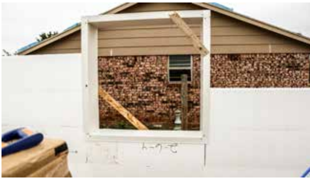
Figure 8.1.2 V-Buck ICF bucking placed into the walls. Notice cross-bracing on corners to ensure it remains square.
