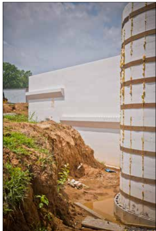
Figure 6.3.2 Brick ledge forms installed at varying heights to support masonry facade above grade.
