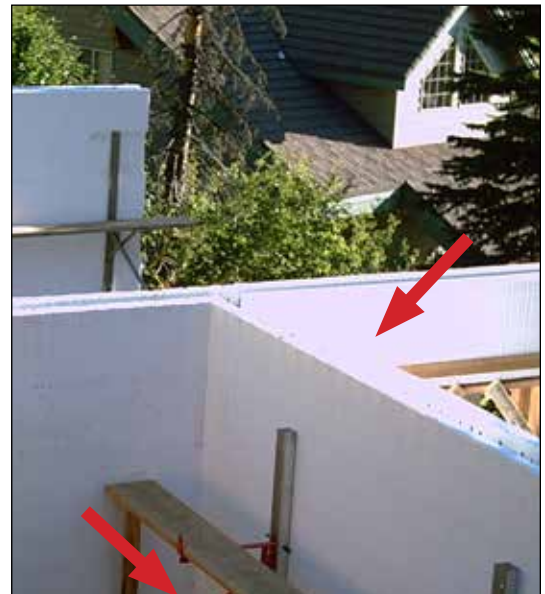
Figure 5.5.9 Intersecting wall opening types.
