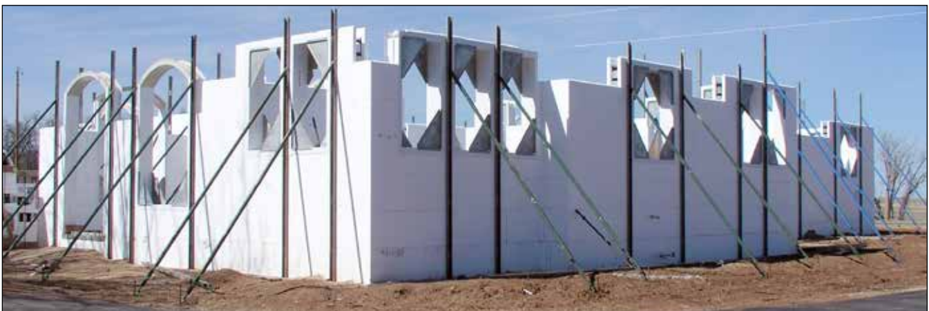
Figure 8.4.2 For larger openings than 3' wide, additional bracing and "bracing legs" (long 2x4 wood legs screwed to the vertical bucks and run to a base plate will help keep your openings straight and plumb during the pour..
