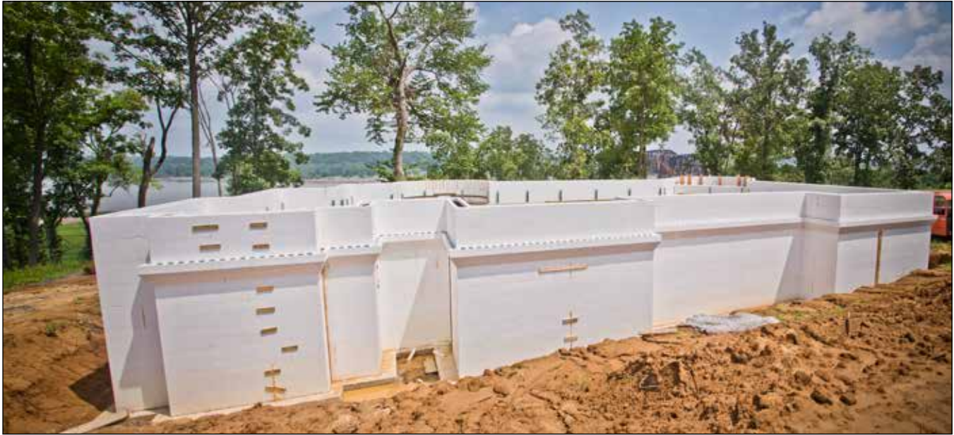
Figure 6.3.1 ICF walkout basement with brick ledge installed to support masonry veneer above grade.
