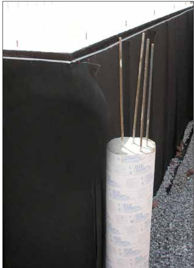
Figure 6.4.9 Basement with pier for footing above. This is done to prevent sagging of footing as the disturbed soil settles.
