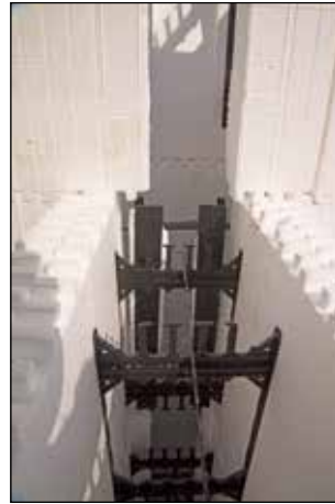
Figure 5.5.6 Intersecting wall opening with wire used to secure webs to intersecting block.
