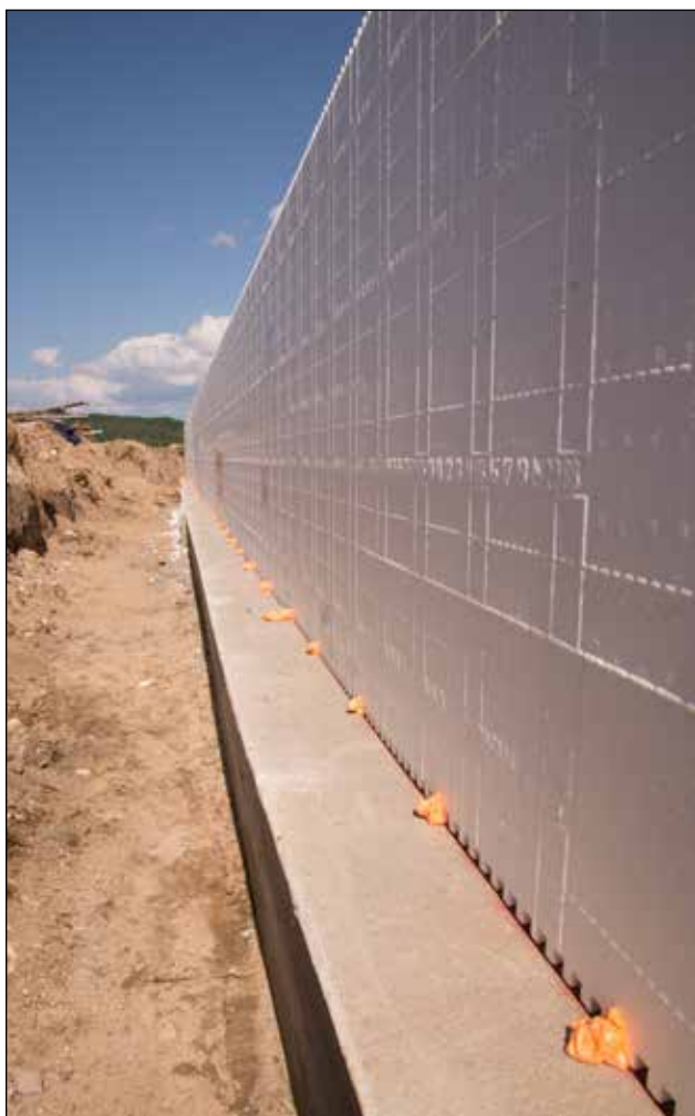
Figure 4.3.2 First two courses leveled and spot glued using foam adhesive. Use small amounts to prevent lifting the wall. Add additional adhesive after spot glue sets if desired.
