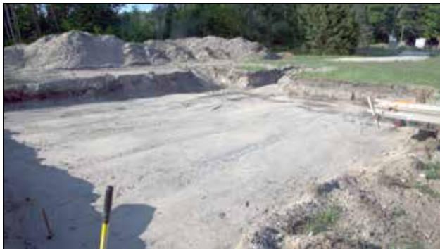
Figure 4.1.4 Excavated Footprint for footings.
