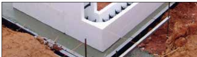
Figure 6.1.5 String lines used to ensure square and ICF form above corner forms locking corner in place until set.
