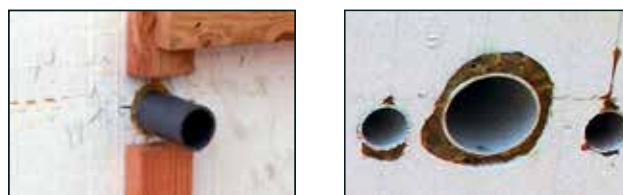
Figure 7.1.5 Add additional strapping if necessary, cut pipes flush after the pour for a seamless finish.
