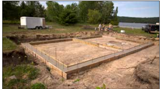
Figure 4.1.8 Place vertical rebar dowels with the correct height to join in the ICF wall.
