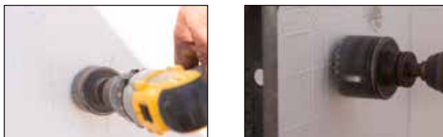
Figure 7.1.2 Drill hole the same diameter as the pipe sleeve to be used.
