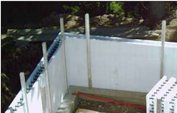
Figure 9.6.3 Minimal Inner Bracing
