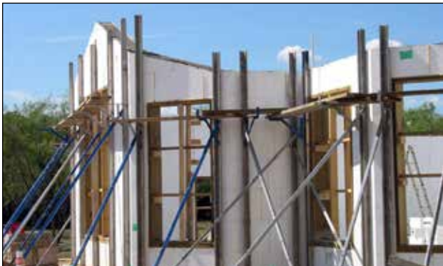
Figure 9.6.2 More Secure Outer Bracing
