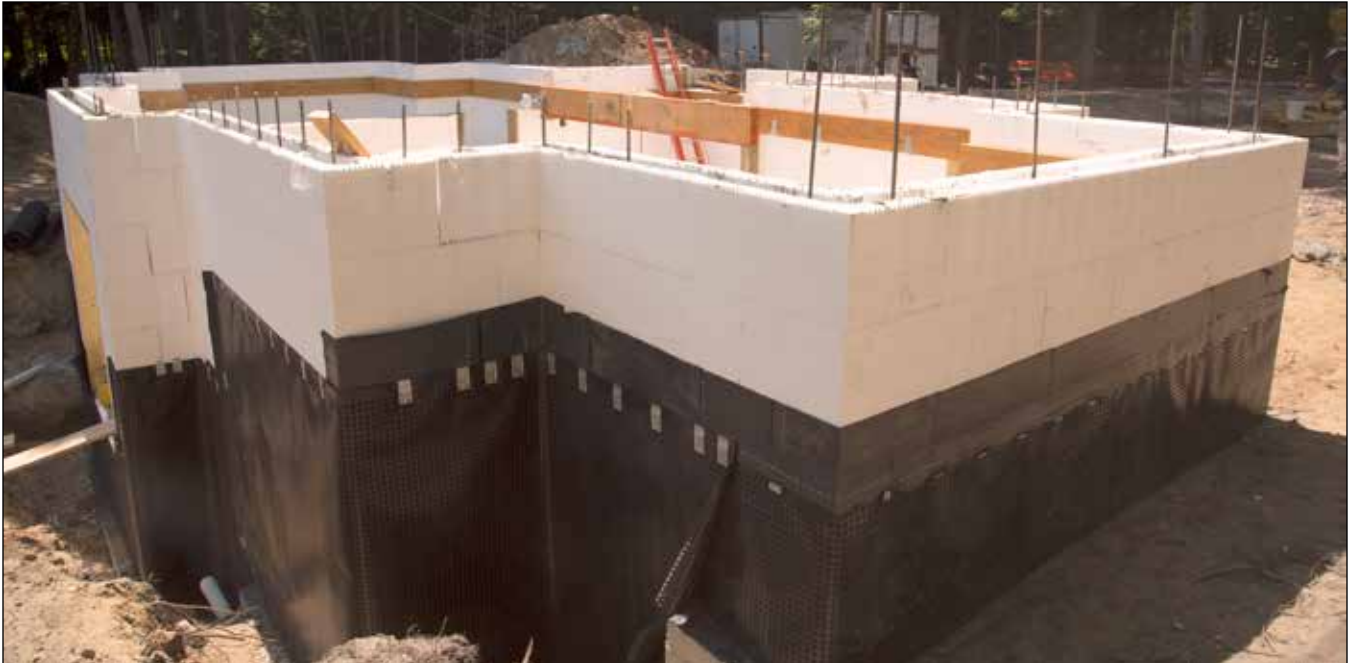
Figure 6.4.1 Below grade ICF walls with Tamko TW-60 peel and stick membrane waterproofing applied and DMX-AG Dimpled Membrane to prevent damage from backfill and provide hydrostatic pressure relief.
