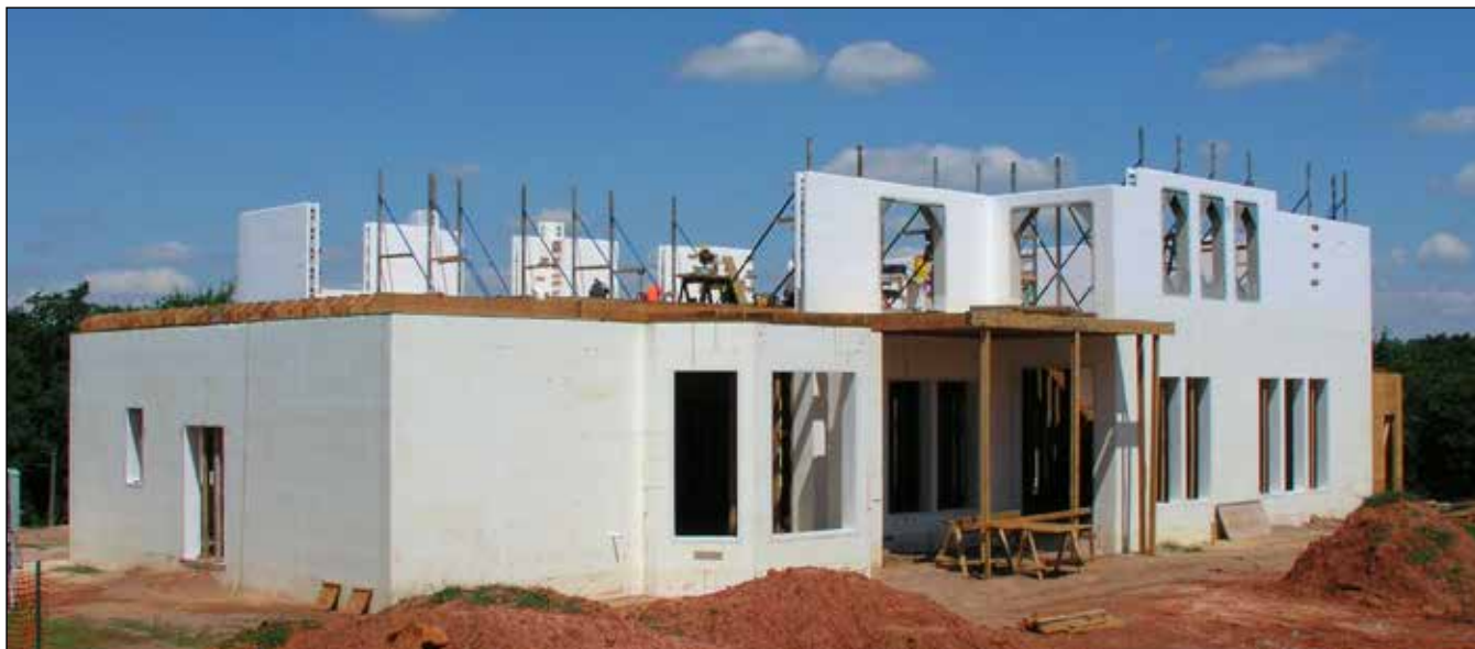
Figure 5.8.1 This partial second story has many openings, steps in height, bulkheads for wood frame attic, and is braced on the inside of the wall.
