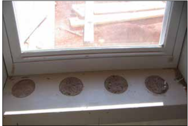
Figure 8.1.4 Fill holes cut into the bottom of a window. Ensure entrained air can escape when pouring a window to prevent any voids.
