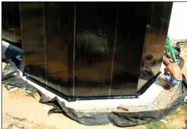
Figure 6.4.3 Installer placing a self-adhesive waterproofing membrane. Notice the 4" of membrane at the bottom of the wall.
