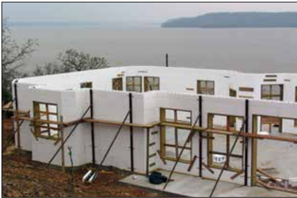
Figure 9.6.1 Minimal Outer Bracing
