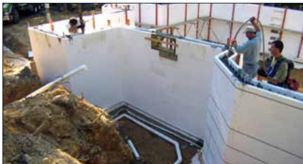
Figure 6.1.2 Standard french drain using slotted PVC pipe:
