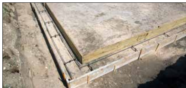
Figure 4.2.2 Formed and reinforced footings ready for pouring.
