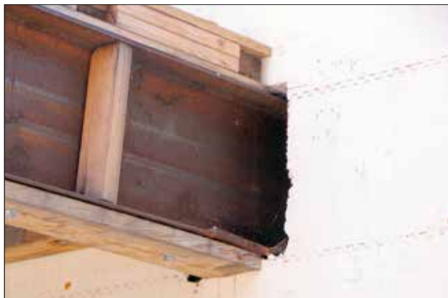
Figure 5.11.1 Steel beam placed in ICF beam pocket.
