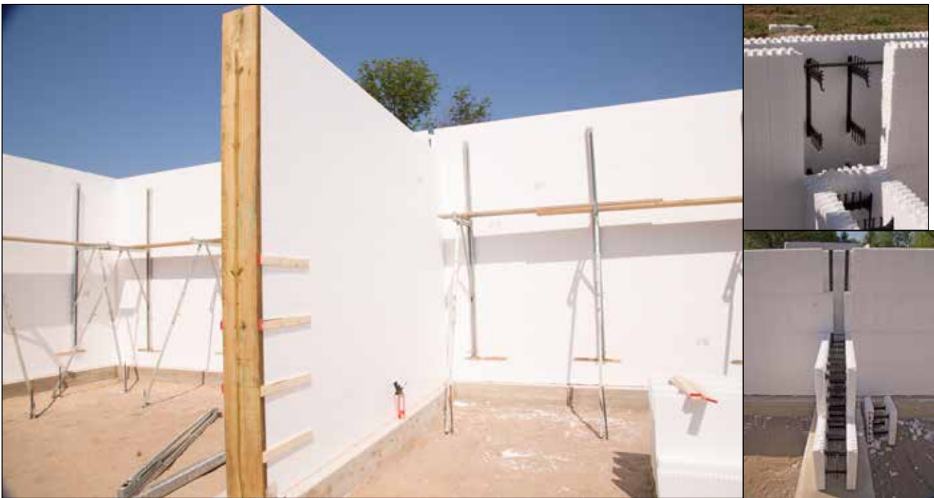
Figure 5.5.1 Intersecting Bulkhead wall with strapping. Figure 5.5.2 (top) Wall intersection opening cut. Figure 5.5.3 intersecting wall opening types.
