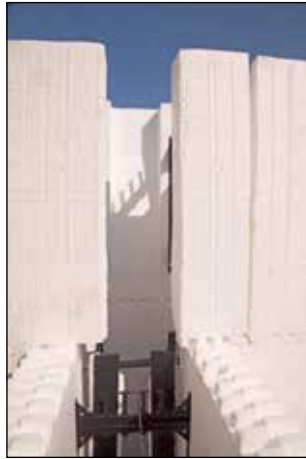
Figure 5.5.5 Intersecting wall opening alternating form placement.
