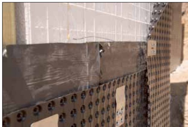
Figure 6.4.6 Waterproofing and air gap membrane is carried at least 1-foot above backfill level. Comply with local codes.
