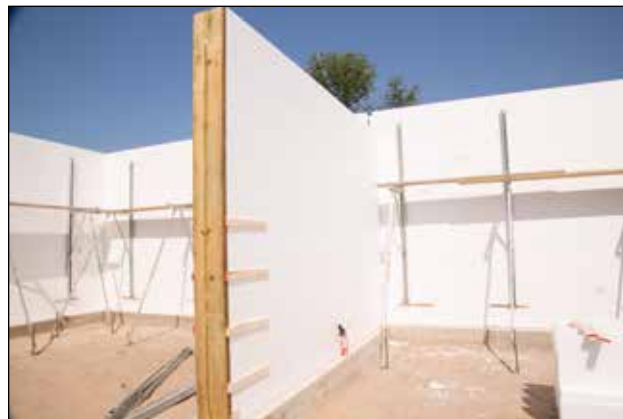
Figure 5.12.1 An end wall, properly braced and strapped prior to installation of bracing & alignment system before concrete pour.
