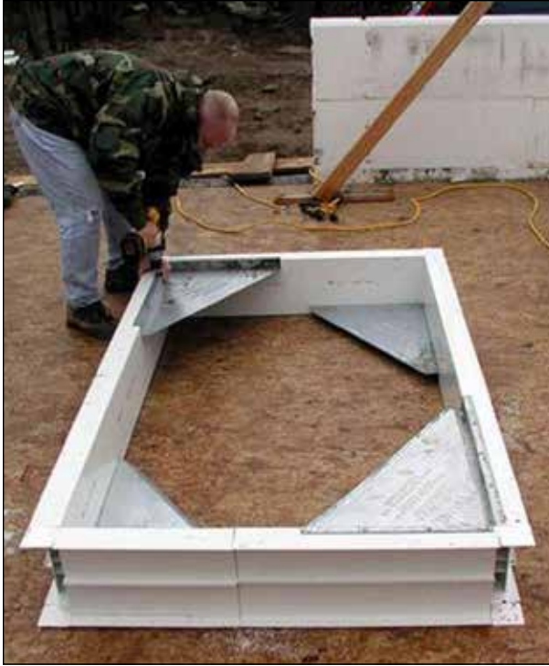
8.2.1 All bucks must be angle braced to keep them square and true.
