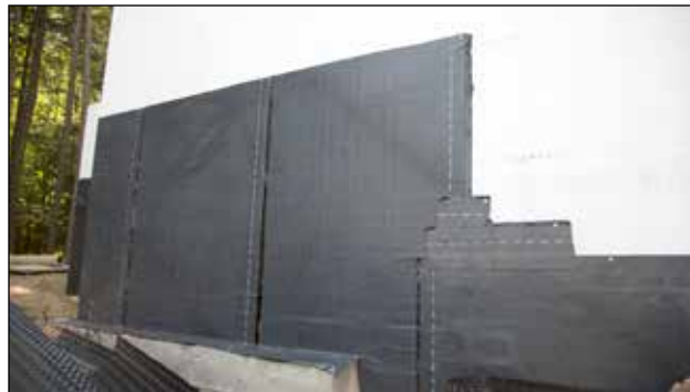
Figure 6.4.4 Peel and stick membrane attached to the ICF wall and sealed to the top of the footing.
