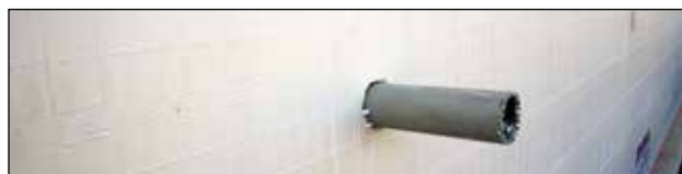
Figure 7.1.4 Secure any space around the pipe sleeve with foam adhesive before the pour.
