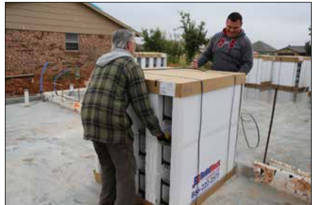
Figure 1.6.3 BuildBlock forms are easily moved around a job site by 1 or two people Drag do not roll to prevent damaging interlock or edges.
