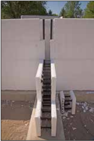
Figure 5.5.4 Intersecting wall opening types.
