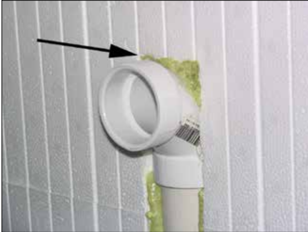
Figure 11.1.7 2" PVC pipe chased into an ICF wall.
