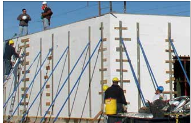
Figure 9.6.5 Ample Outer Bracing with "Scabs" on Non-Factory or Irregular Cut Joints (No Walk Boards)
