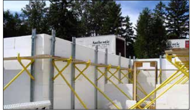
Figure 9.6.4 More Secure Inner Bracing w/ Walk Board
