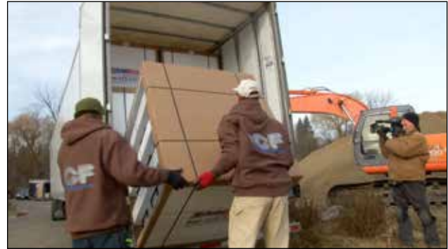
Figure 1.6.2 Unload BuildBlock forms flat to prevent damage to edges and corners.
