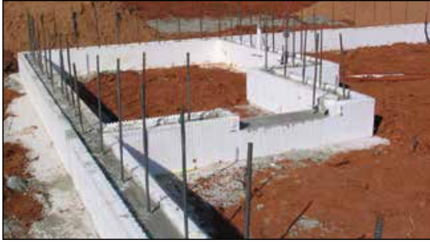
Figure 4.3.4 Wet set BuildBlock ICF stem wall. The first course is square, stacked, and poured. The site is now ready for the slab to be poured. Notice the rebar extending at least 24" vertically and the clean interlocks so the next course can be stacked.
