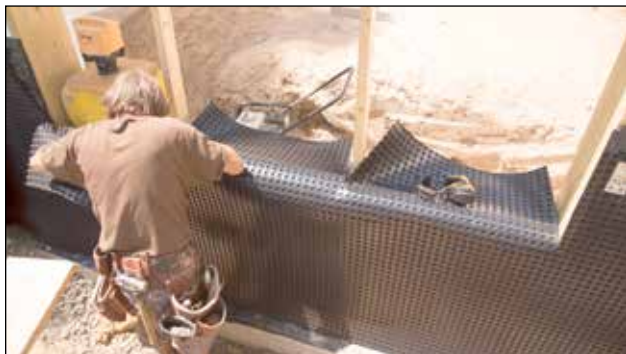
DMX AG membrane attached below large opening.
