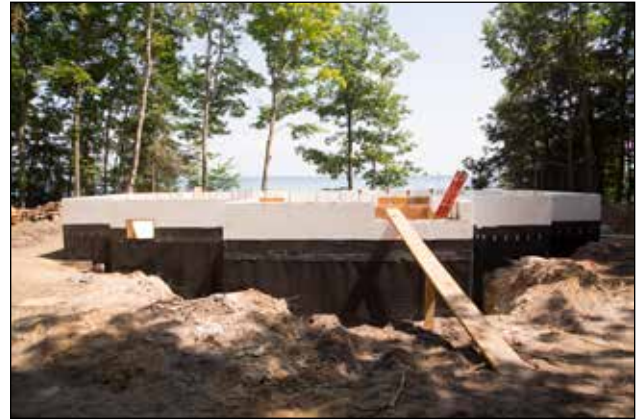
Waterproofing membrane and air gap membranes installed and mechanically attached above final grade level.
