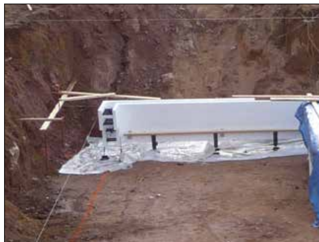
Monopour installation using the Fab Form Monopour System and FastFoot.
