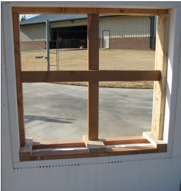
Figure 2.5 Fully cross braced 4040 rough opening.
