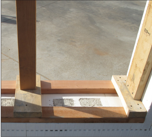
Figure 2.3 Concrete window inspection ports fully filled.
