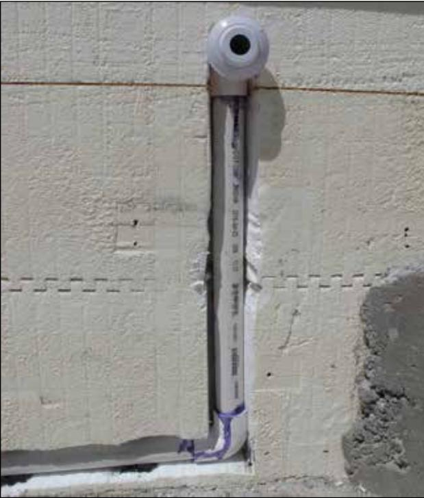
Figure 46: Pool return jet installed.
