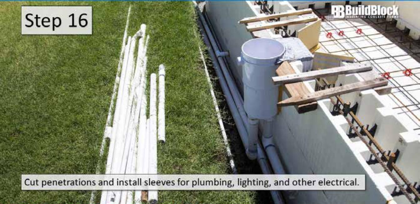
Cut penetrations and install sleeves for plumbing, lighting, and other electrical.
