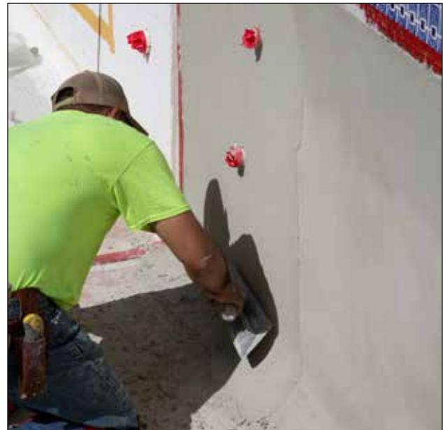
Figure 84: BuildCrete Pool Plaster built up to final thickness and troweled smooth.
