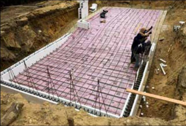
Figure 17: ICF pool with sloped footing.
