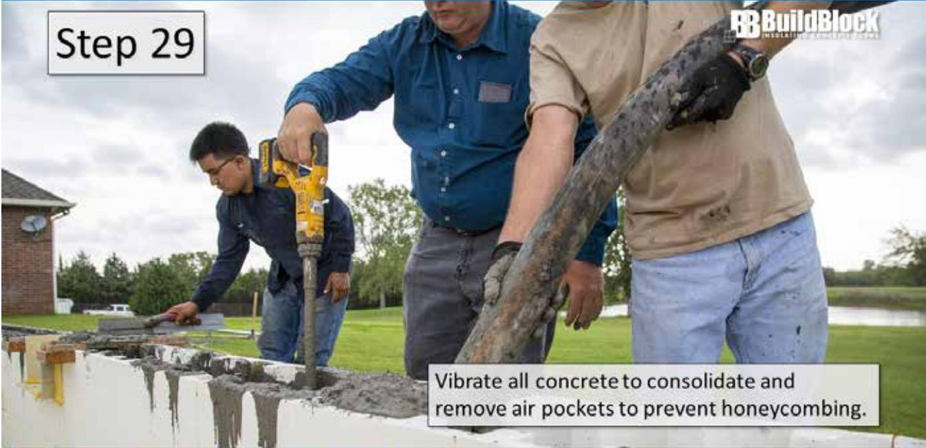
Vibrate all concrete to consolidate and remove air pockets to prevent honeycombing.
