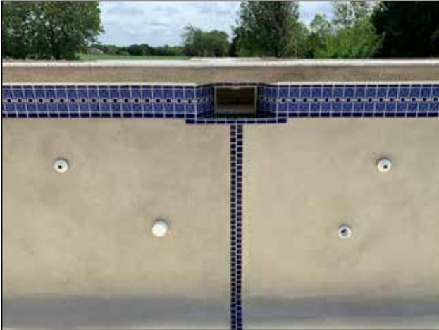
Figure 90: Finished ICF pool skimmer finished with BuildCrete Pool Plaster and tile.
