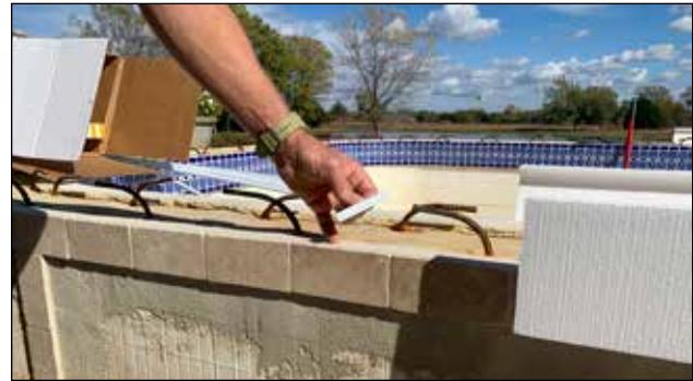
Figure 69: The tile track provides a break between the poured coping and tile to prevent any damage from expansion and contraction.
