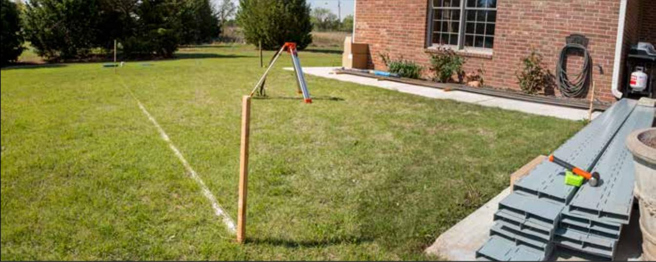
Figure 9: Excavation area marked and benchmark established.
