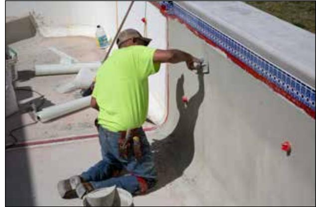
Figure 83: BuildCrete Pool Plaster built up to final thickness and troweled smooth.
