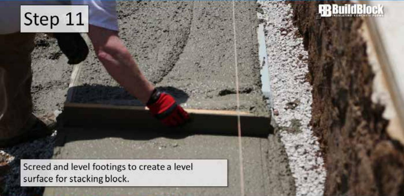
Screed and level footings to create a level surface for stacking block.
