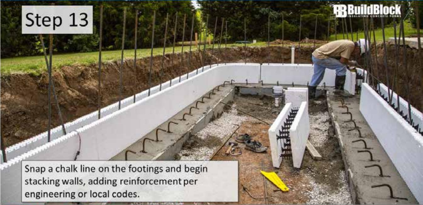
Snap a chalk line on the footings and begin stacking walls, adding reinforcement per engineering or local codes.
