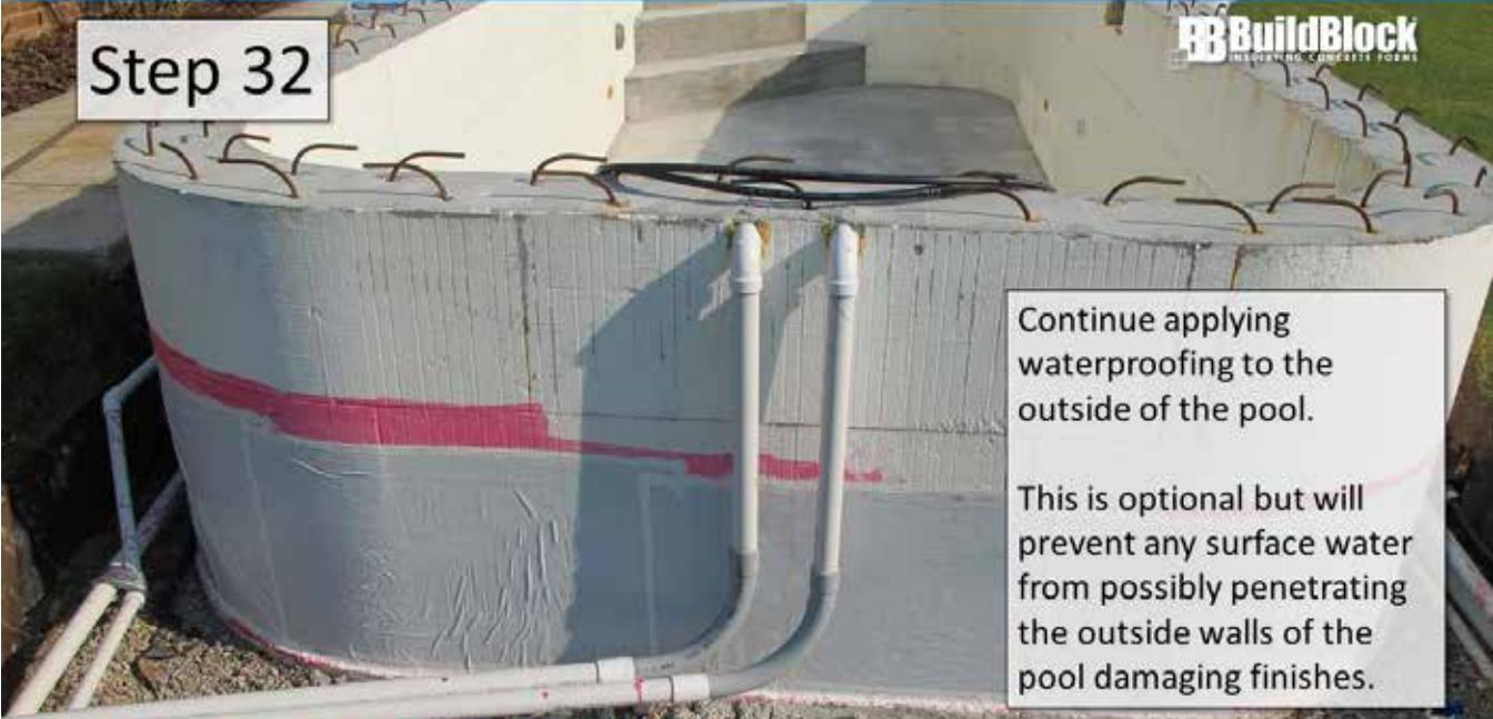
Continue applying waterproofing to the outside of the pool.
