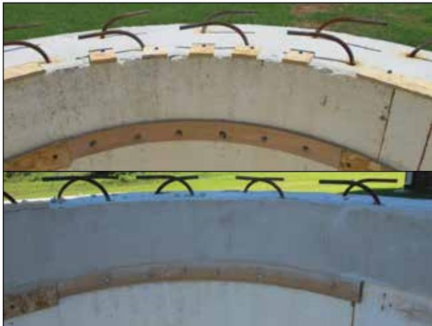
Figure 60: Base installed on top and bottom of curved form to ensure level for tile.
