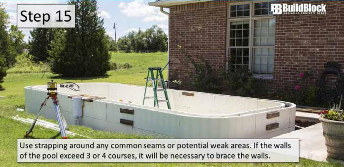
Use strapping around any common seams or potential weak areas. If the walls of the pool exceed 3 or 4 courses, it will be necessary to brace the walls.
