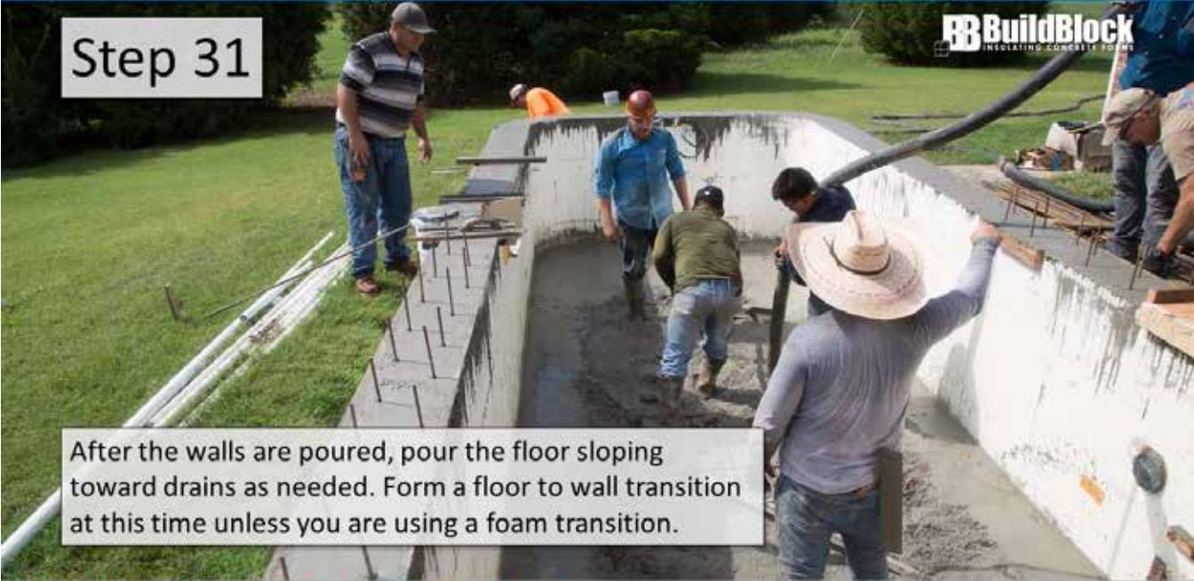
After the walls are poured, pour the floor sloping toward drains as needed. Form a floor to wall transition at this time unless you are using a foam transition.
