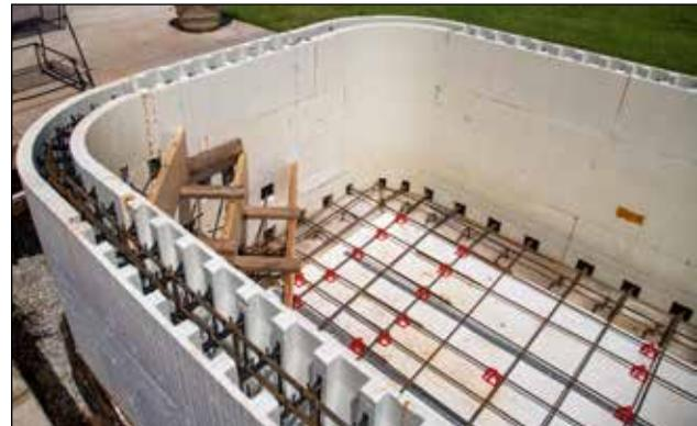
Figure 31: ICF pool floor reinforcement tied into wall reinforcement provides additional strength.
