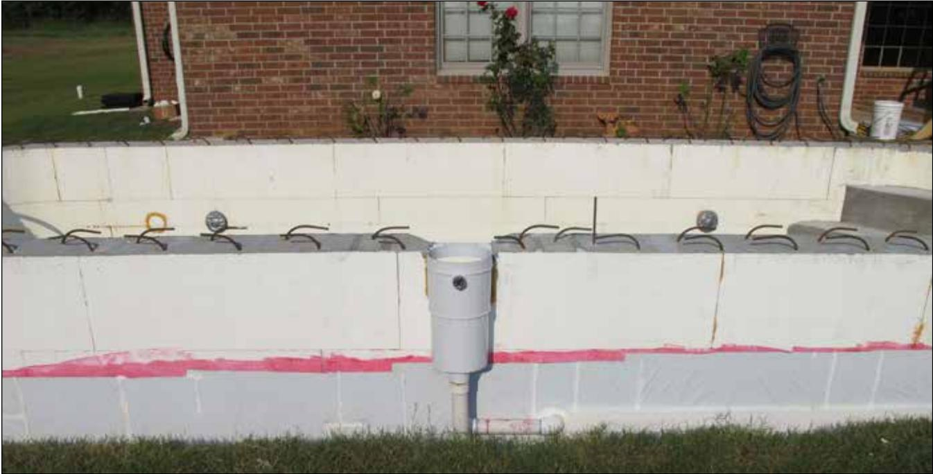
Figure 52: ICF pool with walls poured and waterproofed below grade. This pool uses Form-A-Drain an integrated stay-in-place footing form and perimeter drainage system.
