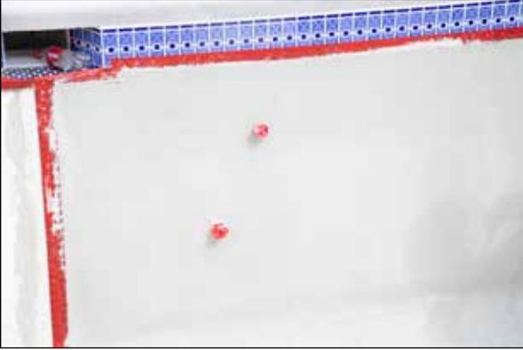
Figure 86: BuildCrete Pool Plaster built up to final thickness and troweled smooth.
