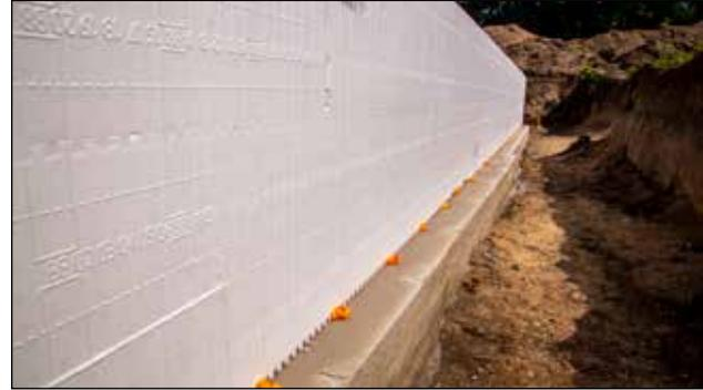
Figure 28: Two courses of ICF wall stacked, shimmed and trimmed, spot glued in place.
