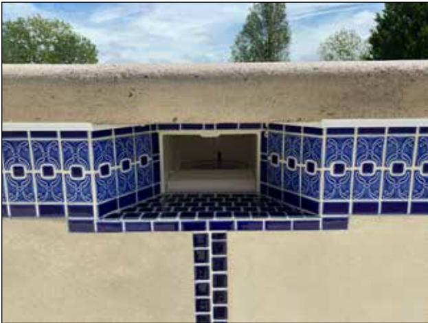
Figure 91: Finished ICF pool skimmer finished with BuildCrete Pool Plaster and tile.
