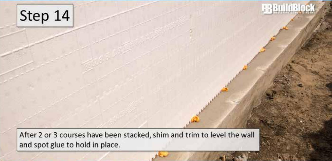
After 2 or 3 courses have been stacked, shim and trim to level the wall and spot glue to hold in place.
