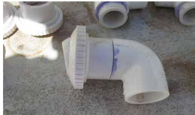
Figure 44: Pool return jets premade to correct length to match with pool finish.
