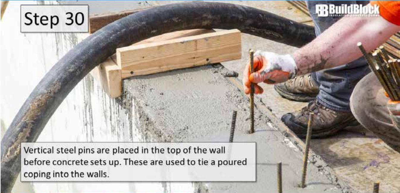
Vertical steel pins are placed in the top of the wall before concrete sets up. These are used to tie a poured coping into the walls.
