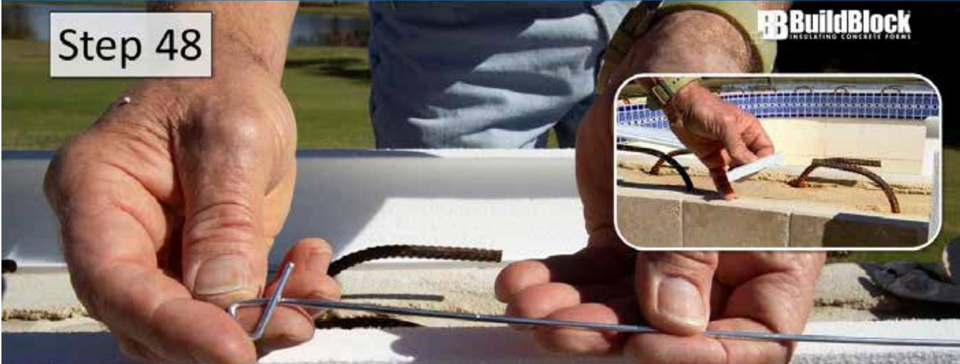
Set the shaped coping using the plastic spacer and the adhesive on the forms. The plastic spacer ensures concrete does not bond to the top of the tile and allows for expansion and contraction. Tie forms to rebar using breakaway metal ties.
