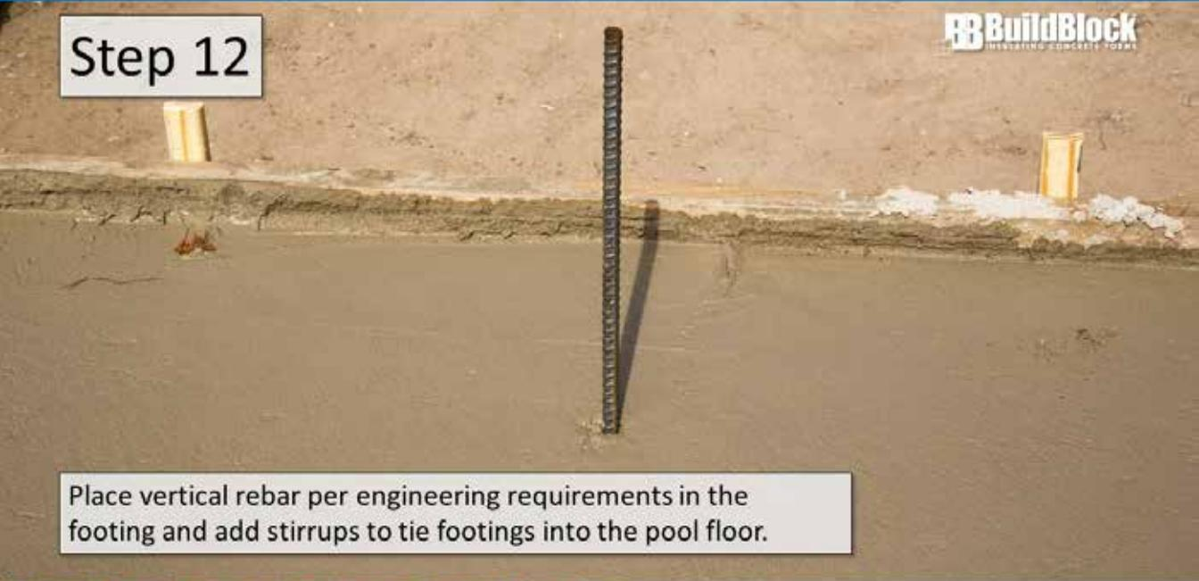
Place vertical rebar per engineering requirements in the footing and add stirrups to tie footings into the pool floor.
