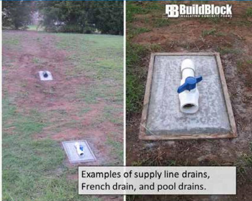
Examples of supply line drains, French drain, and pool drains.
