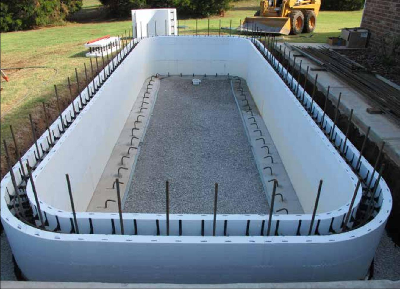
Figure 24: ICF pool walls stacked with reinforcement.
