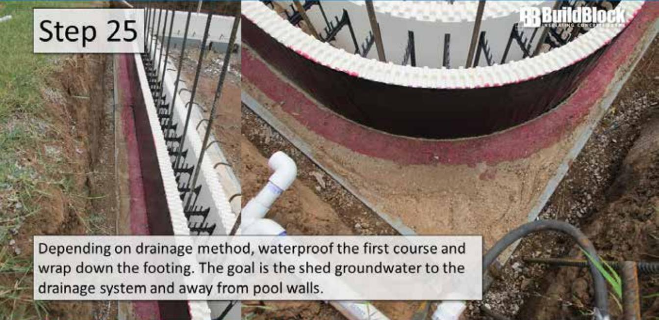
Depending on drainage method, waterproof the first course and wrap down the footing. The goal is the shed groundwater to the drainage system and away from pool walls.
