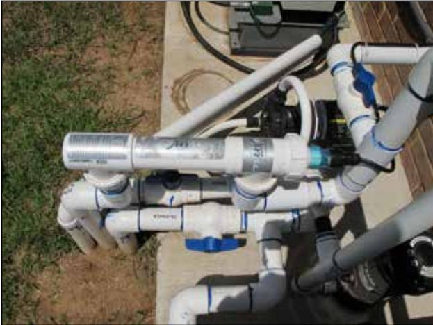
Figure 97: Make sure all plumbing is secured and protected against the environment and is accessible for maintenance as needed.
