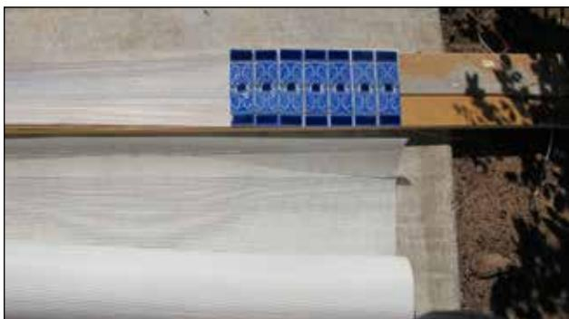
Figure 61: Use a template to cut the mesh for the BuildCrete Pool Plaster.
