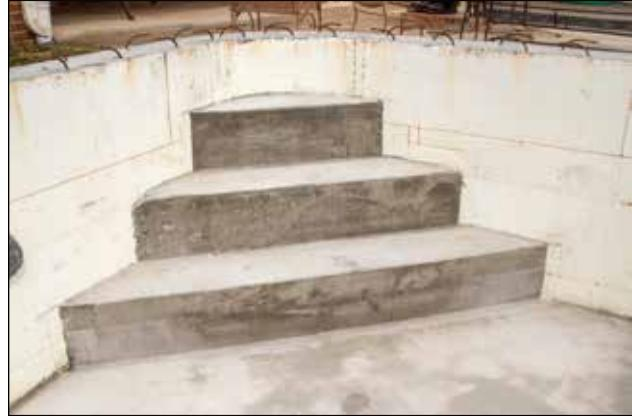
Figure 34: ICF pool steps poured with forms stripped.
