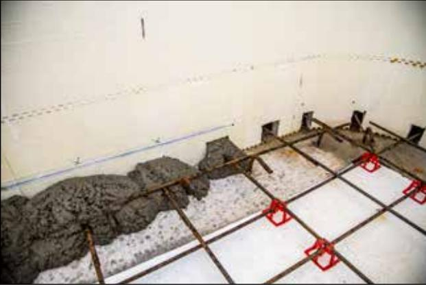
Figure 51: Pouring ICF pool walls.
