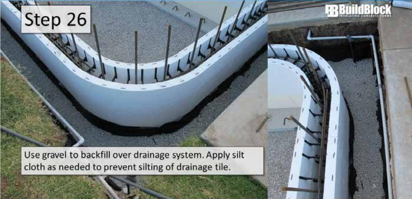
Use gravel to backfill over drainage system. Apply silt cloth as needed to prevent silting of drainage tile.
