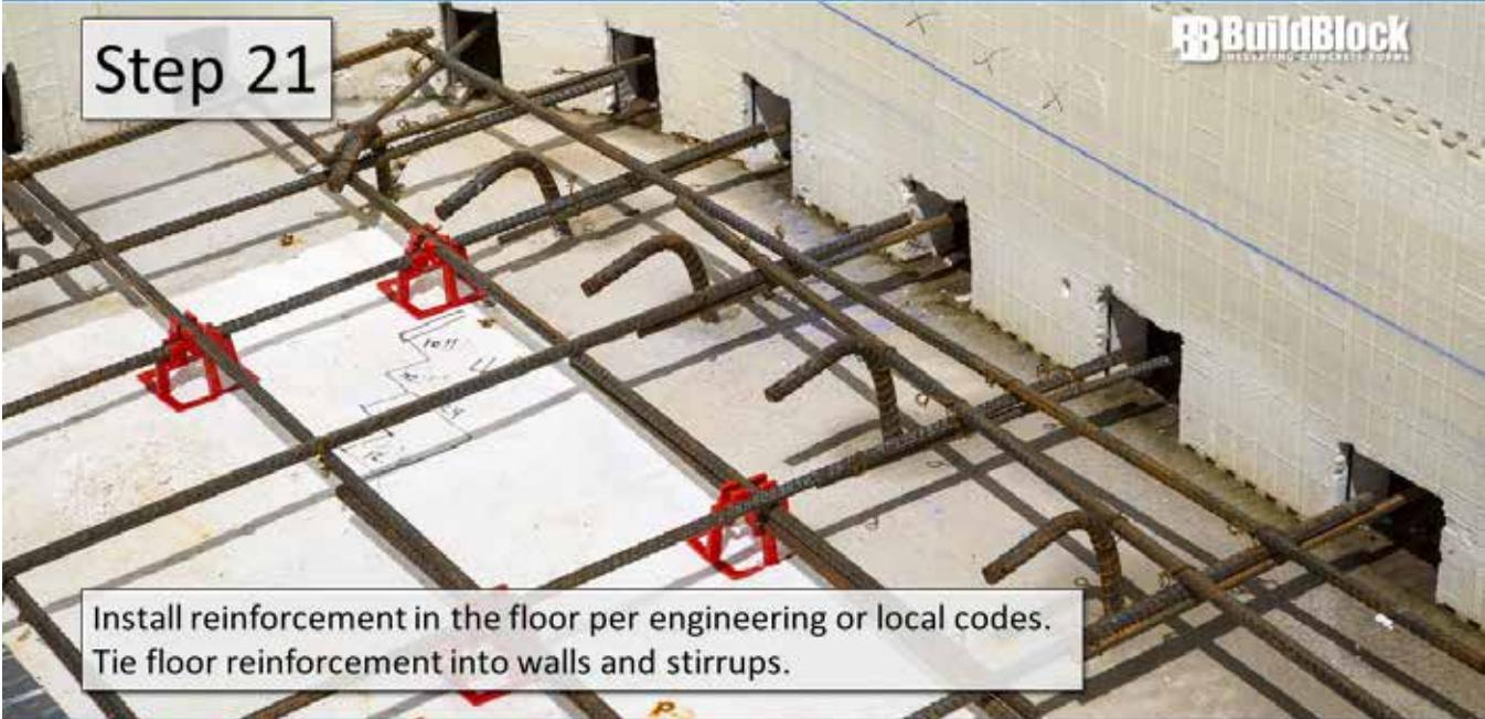
Install reinforcement in the floor per engineering or local codes. Tie floor reinforcement into walls and stirrups.
