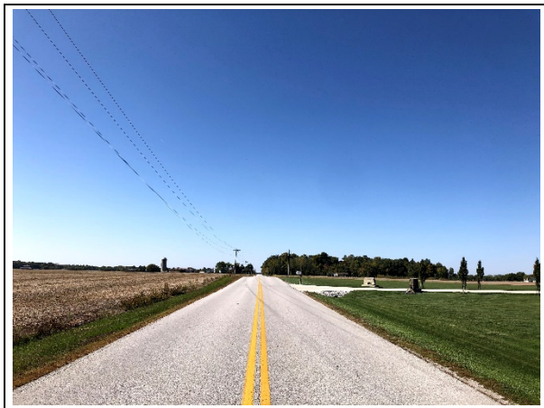
Photo 21. National Road halfway between Bowsher Rd and railroad crossing, view west
