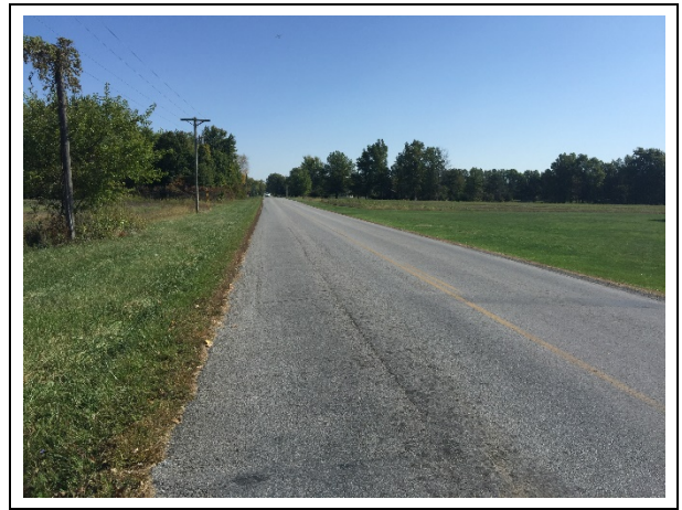
Photo 2. Fort Amanda Rd, at S. Kemp Rd, view east
