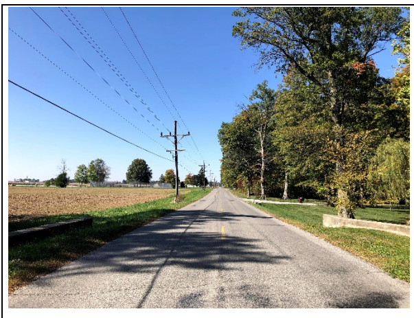
Photo 5. W. Breese Rd, 0.25 mile from SR 501 at culvert, view west
