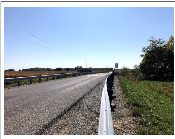
Photo 17. Load rated bridge on S. Kemp Rd, north of Hume Rd.
