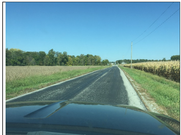
Photo 16. S Kemp Rd at Hume Rd at bend, view north
