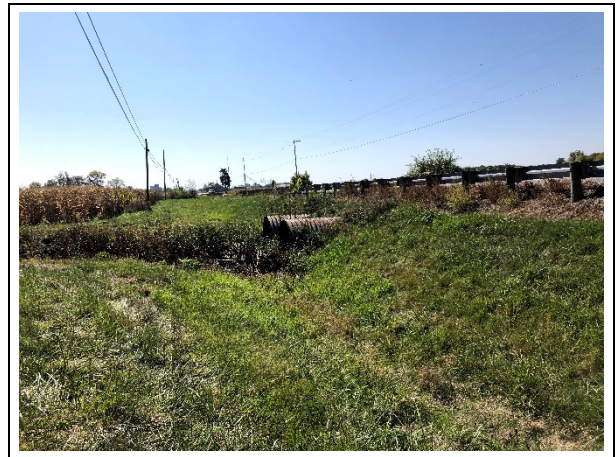
Photo 10. SR 501 culvert at Two Mile Creek, east side (view west)
