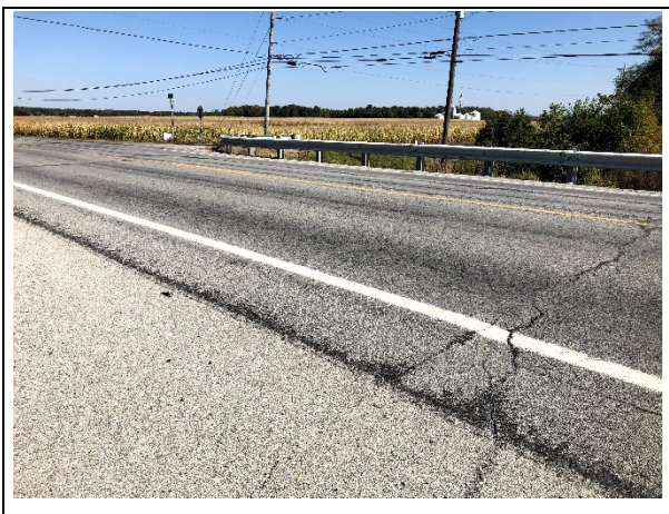
Photo 11. SR 501 at box culvert at Bowsher Rd., view west
