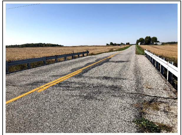
Photo 14. Hume Rd, at Two Mile Creek, view west
