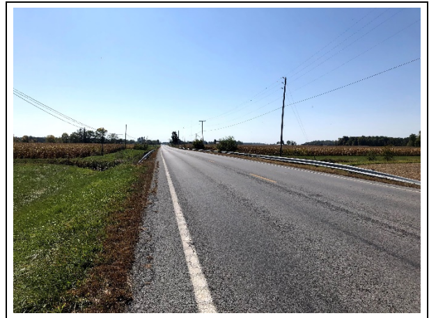
Photo 8. SR. 501, 0.5 mile from W. Breese Rd, at bridge, view south
