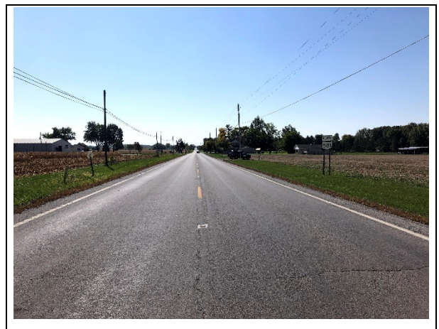
Photo 6. SR 501, at W. Breese, view south
