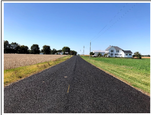
Photo 19. Zerkle Rd at S Kemp Rd, view west
