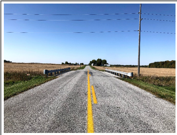
Photo 13. Hume Rd, at Two Mile Creek, view west
