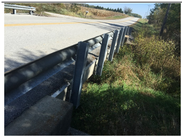
Photo 23. National Rd east of Bowsher Rd, view east
