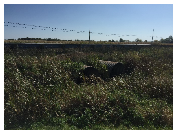
Photo 9. SR 501 culvert at Two Mile Creek, west side (view east)
