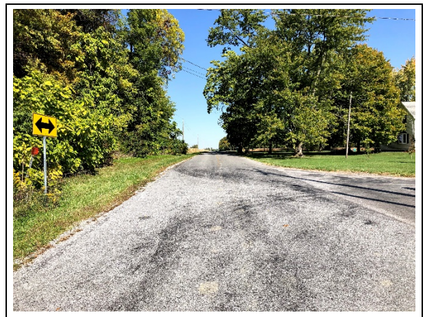
Photo 4. S. Kemp Rd at W. Breese Rd, view north
