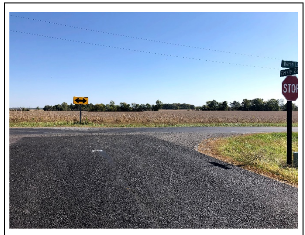
Photo 18. Zerkle Rd and S. Kemp Rd intersection, view east
