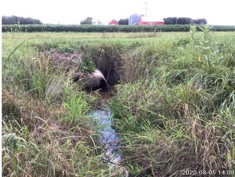
Photograph 47. View of Stream 11. Photograph taken facing downstream, south.
