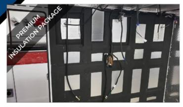
The industry's most efficient insulation package, using state of the art refrigerator technology, is engineered with polyurethane closed-cell insulation, sealed inside the wall structure, and a thermal barrier covers all metal surfaces to limit heat exchange from the exterior to the inside module. It also provides a clean, durable, environmentally safe insulation with pre-engineered service accessibility.
