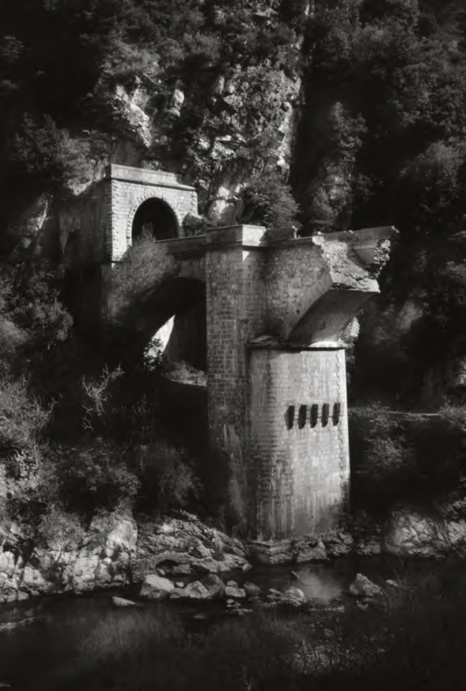
Bombed Railway Bridge, Former Yugoslavia
