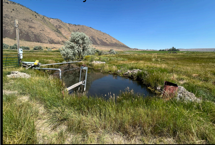
Summer Lake Pump & Pipeline Upgrade for Water Efficiency & Wetland Habitat
