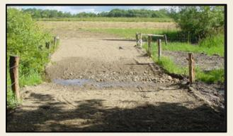
Hardened crossings and water access points are coarse gravel pads that provide livestock secure footing for crossing a stream or for drinking.
