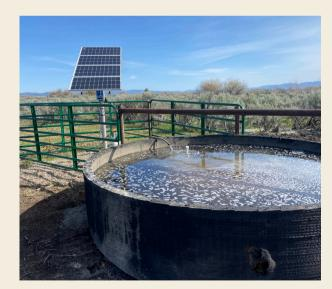
**Offsite water** can be developed by installing solar, hydraulic ram or conventional pumps; developing springs, wells, or guzzlers; and piping water to troughs.
