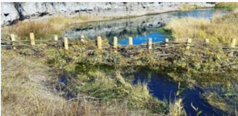
Camas Creek Beaver Dam Implementation - Coyote Moon LLC set over 400 posts to support 14 structures (Oct)
