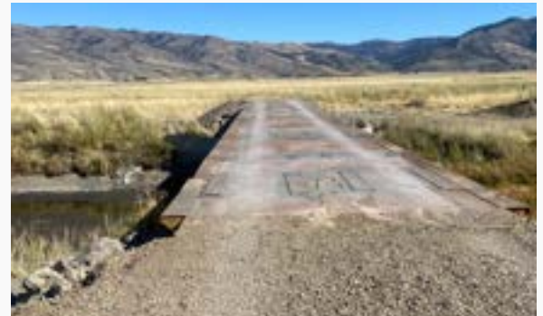
Thomas Creek Amsbaugh Diversion Railcar Bridge, placed to help remove stop panels - Dog Lake Construction (Oct)
