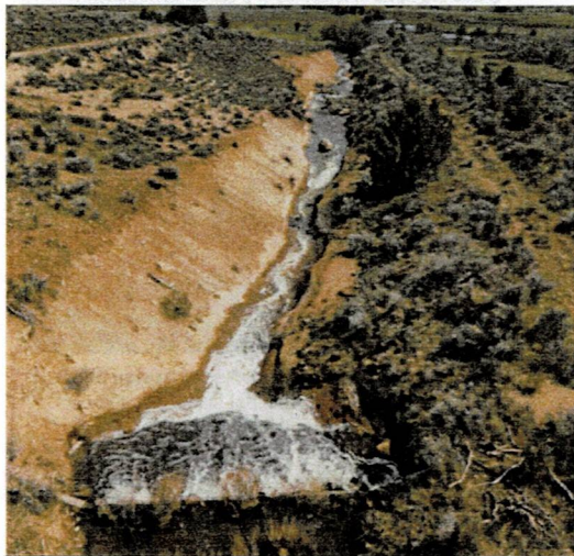
Photo of existing spill way that will be reconstructed to provide a roughened channel for fish to travel up and into Juniper Reservoir.
