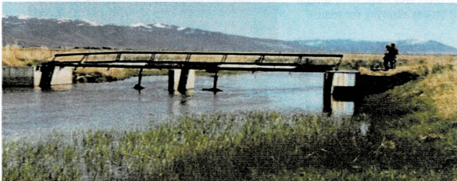
Photo of the current diversion structure with a dated and non-functioning fish passage to the right. Design plans include a bypass channel around the diversion for fish passage.
