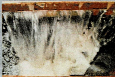
One of the 67 leaky headgates on the canal system.
