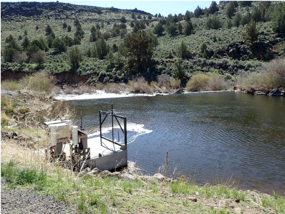
Photograph of the MC Diversion showing fish bypass box culvert and diversion dam.
