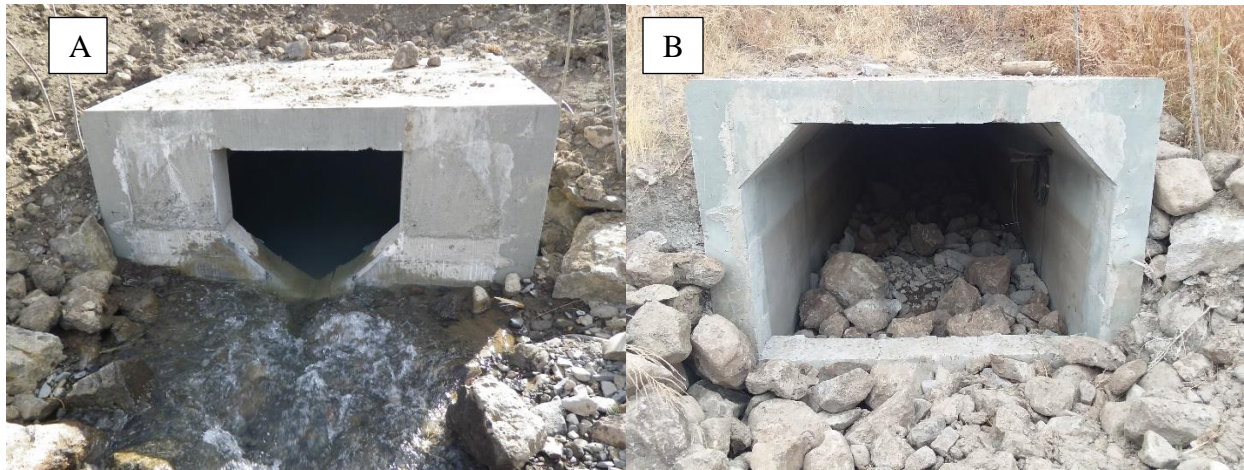
Figure 3. Photos of MC bypass culvert showing original V-notch weir (A) and modified downstream opening (B).
