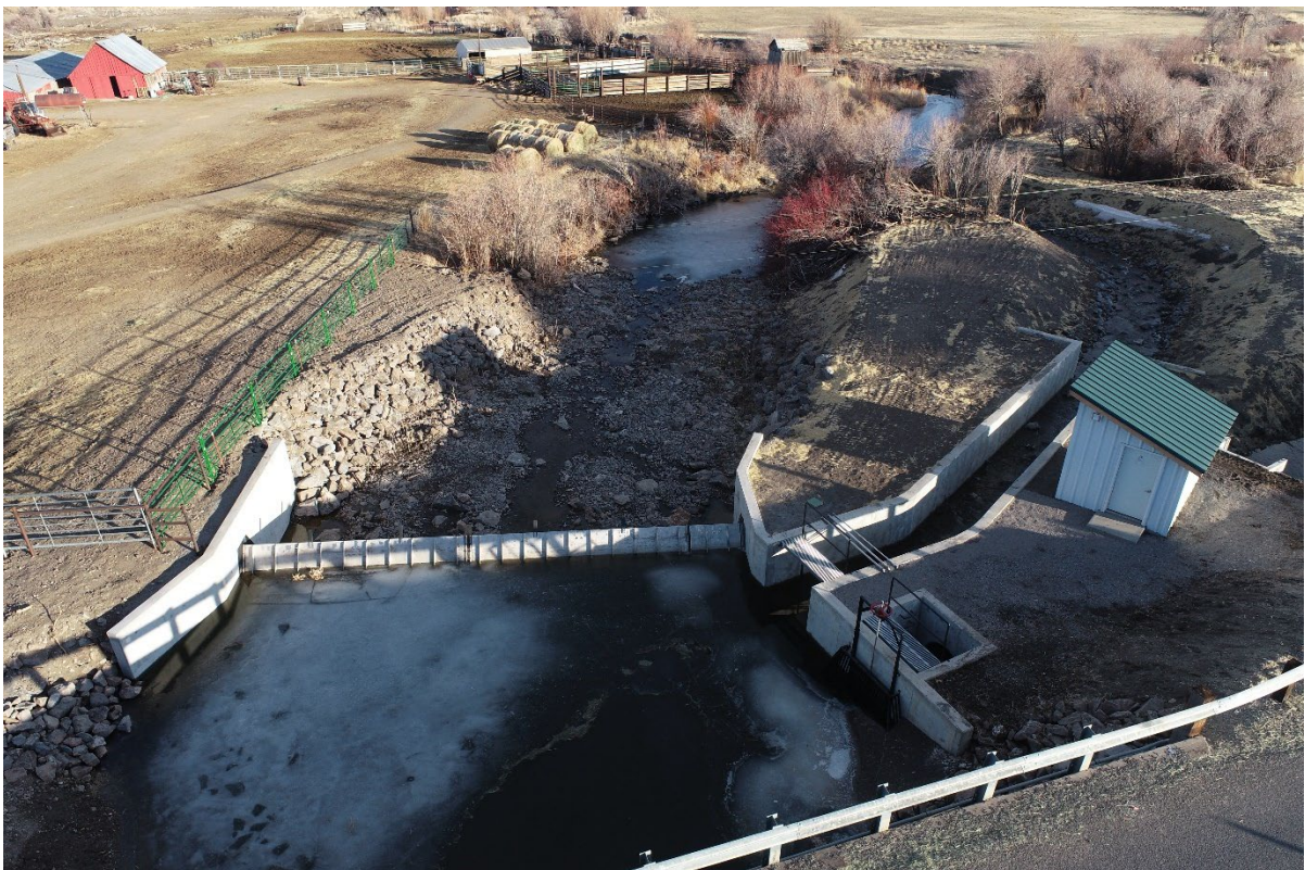
Obermeyer weir and fishway channel at Plush-Town Diversion on Honey Creek. Photo credit: Troy Brandt, River Design Group
