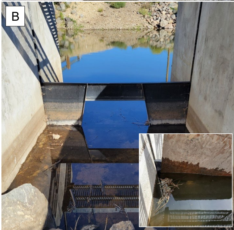
Appendix Figure 2. Photos of partially opened Obermeyer weir during spring of 2022 (A) and metal stoplog with orifice at upstream end of the fishway channel (B) at Plush-Town Diversion. Inset photo in photo B show orifice blocked with plywood.
