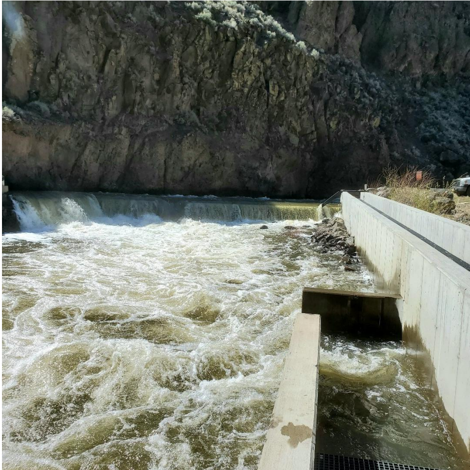
O’Keeffe Diversion Dam and fish ladder on Deep Creek during high flow in 2025 (740 cfs)
