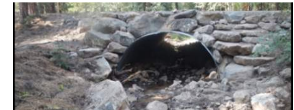
Pipe Arch Culvert with stream simulated design within the interior. Provides free upstream and downstream movement
