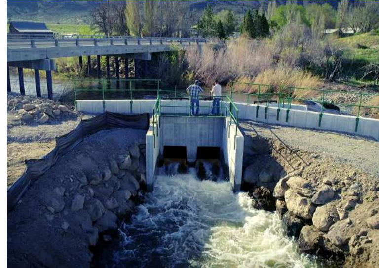
Deep Creek Town Diversion and Fish Passage Project 2019
