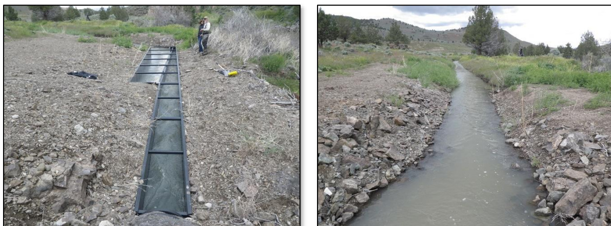
Figure 6-3. The FCA fish screen on the Dyke diversion irrigation canal (left) and the open canal downstream of the screen (right).
