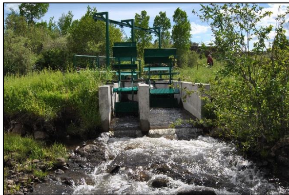
Figure 5-6. Example paddle wheel-driven rotary drum screens at the O'Keeffe diversion on Deep Creek (left) and the Taylor diversion on Honey Creek (right).
