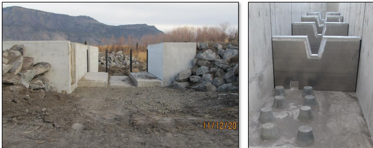
Figure 6-7. The reconstructed Rookery diversion weir on lower Honey Creek (left), includes wooden cross-walls, a 9-inch square orifice in each cross-wall, and artificial boulders on the ladder floor to reduce velocities (right).
