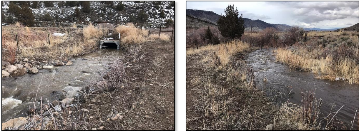
Figure 6-5. Upstream (left) and downstream (right) views of the MC bypass channel in March 2019.
