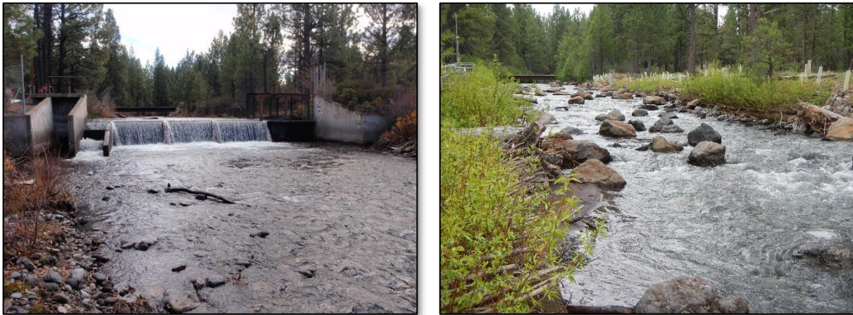
Figure 5-3. An irrigation diversion weir on Whychus Creek near Sisters, Oregon before (left) and after (right) the construction of a roughened channel.
