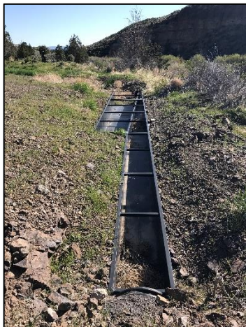
Figure 5-9. The 6.25 cfs modular FCA screen at the Dyke diversion on Twentymile Creek (left) and the 150 cfs custom fabricated FCA screen at the Three Sisters Irrigation District diversion on Whychus Creek near Sisters, Oregon (right).
