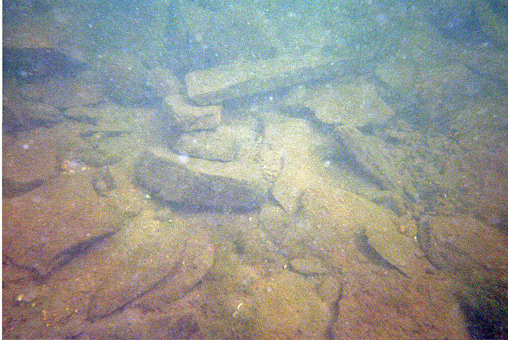
Remaining Loose Foundation
