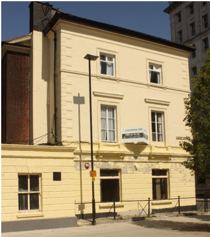
Figure 15 South elevation of the main range.
