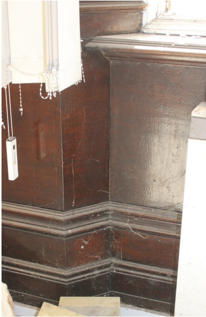
Figure 21 Detail of the panelling to dada level and below the windows.
