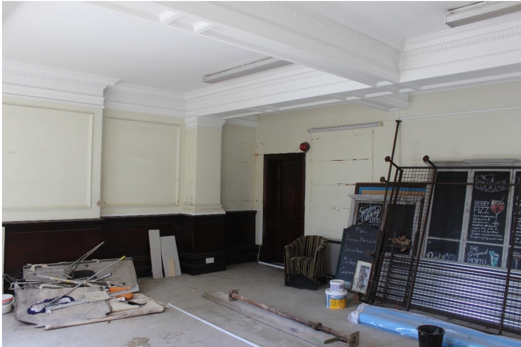
Figure 19 The southern room of the main range, facing north-west.
