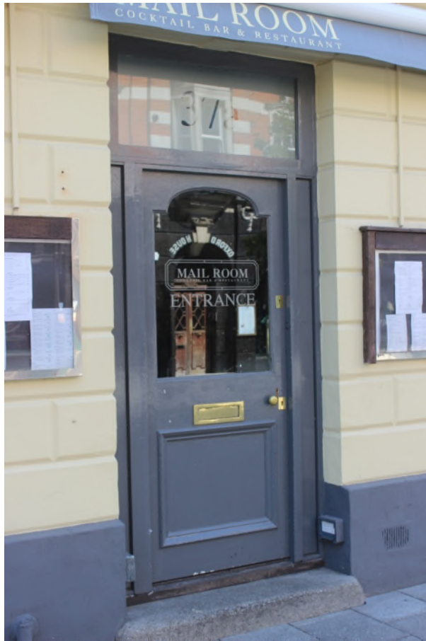
Figure 24 Inserted door replacing a window in the north, Oxford Street elevation.
