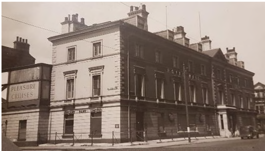
Figure 12 Postcard of the Royal Mail Lines offices c.1940-50, south and east elevations.
