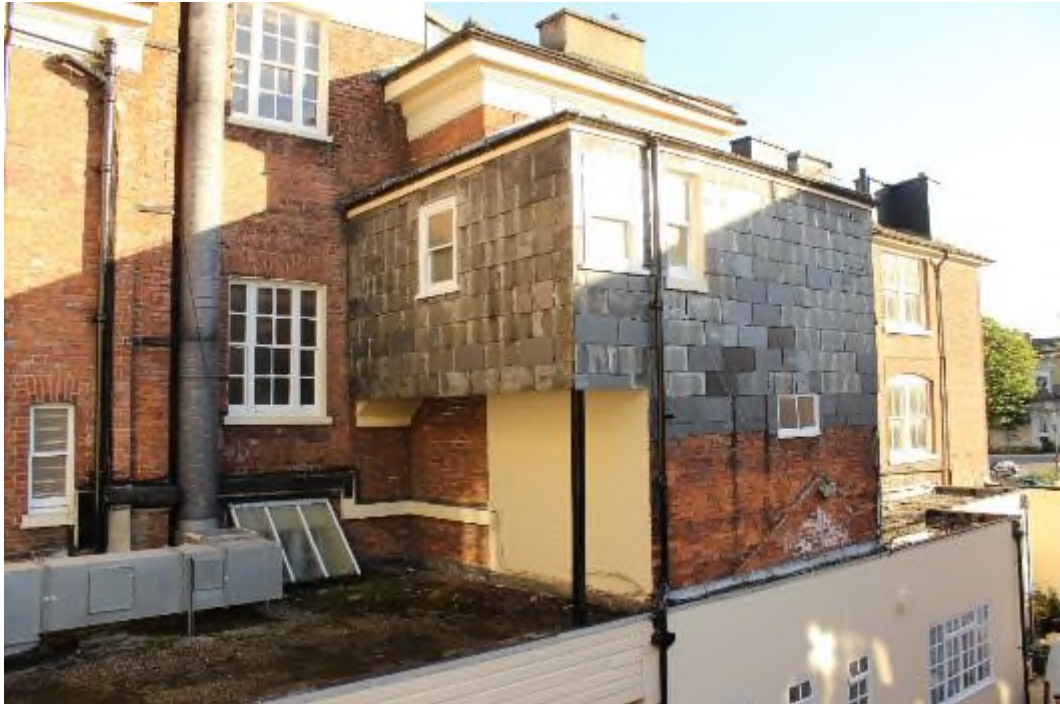
Figure 17 Rear elevation of the Terminus Terrace range, central part.
