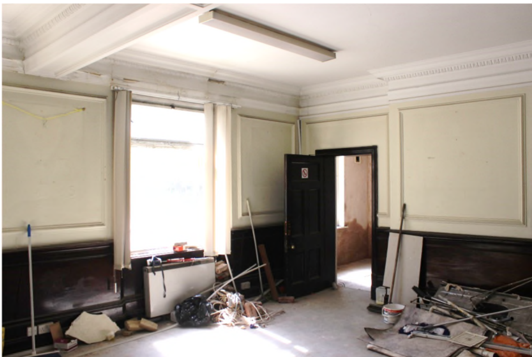
Figure 20 The southern room of the main range, facing south-west.
