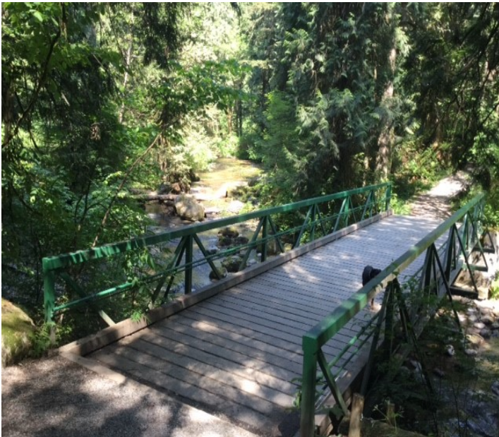
Bridge at the North Fork of Kanaka Creek.
