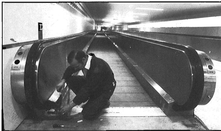
Above: The site team at Heathrow London Airport Below: Mick Corley fitting a handrail brush box
