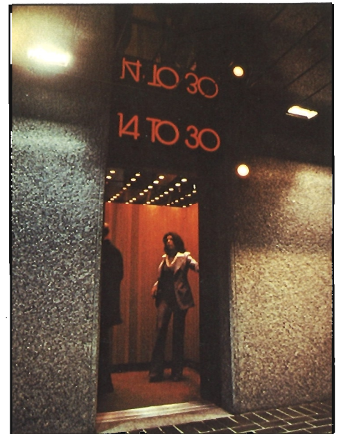
Below. The Otis vertical transportation system includes 20 double-deck elevators that serve two floors simultaneously
