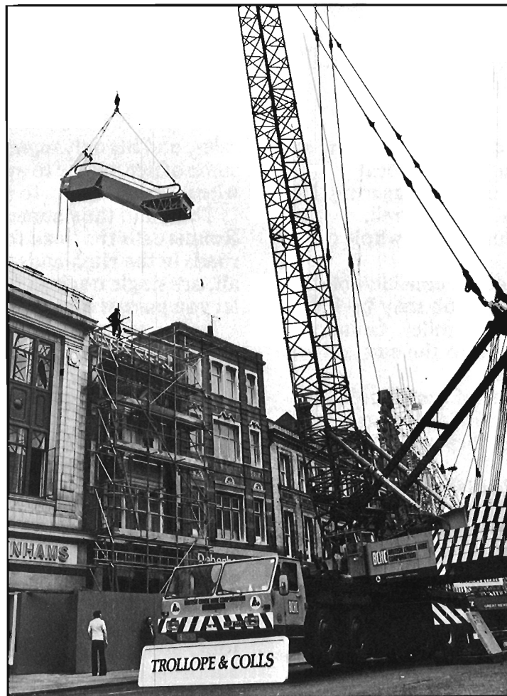
One of six Otis escalators rising high as it goes into Debenhams store at Reading. The photograph is by Alec Goatley, Bristol construction supervisor
