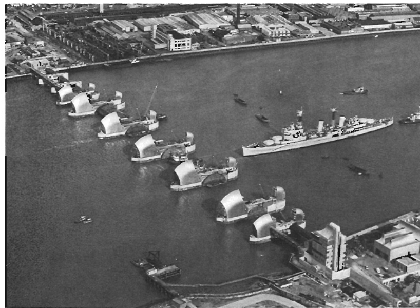
Thames Barrier equipped by Evans.
