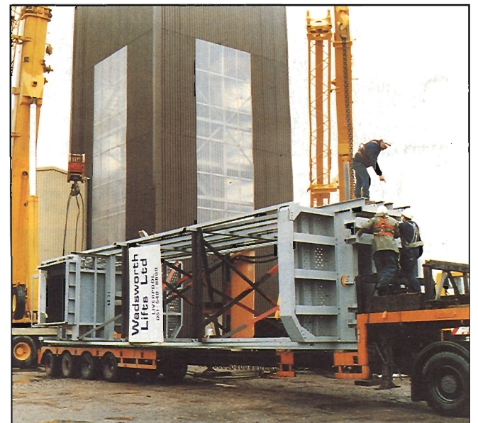
Moving into position.
