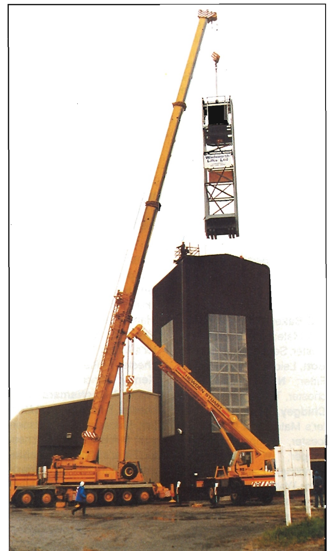
Feeding the car down on to the guides.
