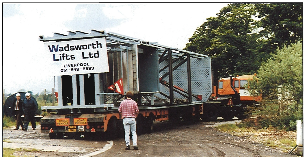
Reversing on to the site. The low loader has steerable rear wheels.
