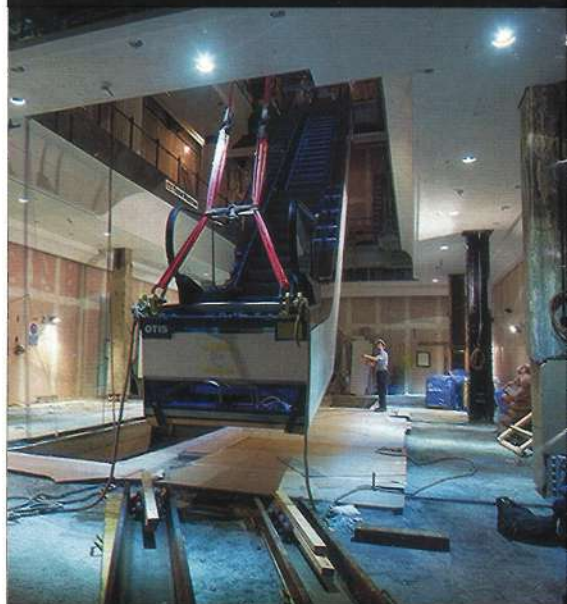
One of the ground-to-first floor escalators being transferred across the well.
