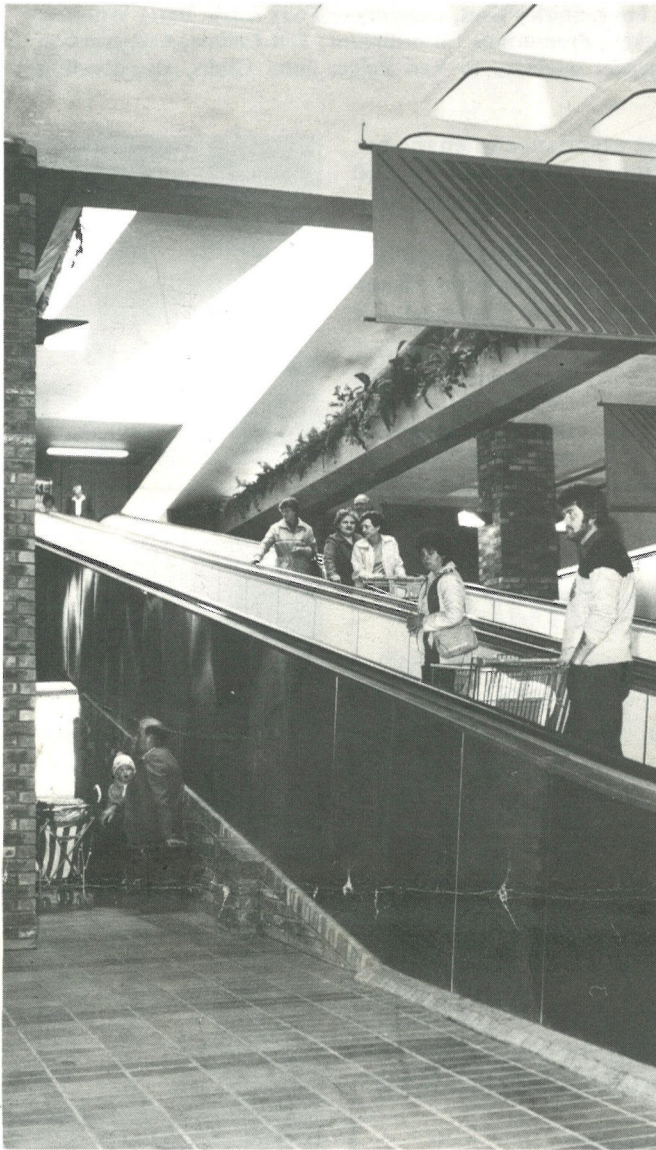
Above, the two travolators are in a mall outside the entrance to the store. Below left, the trolley wheels lock into the tread of the travolators during the ride.
