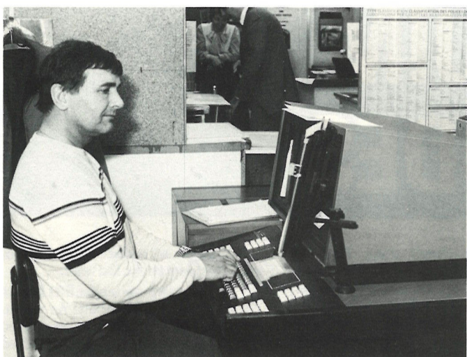
Fred is a compositor. This machine sets type electronically and photographically. There is no metal type
