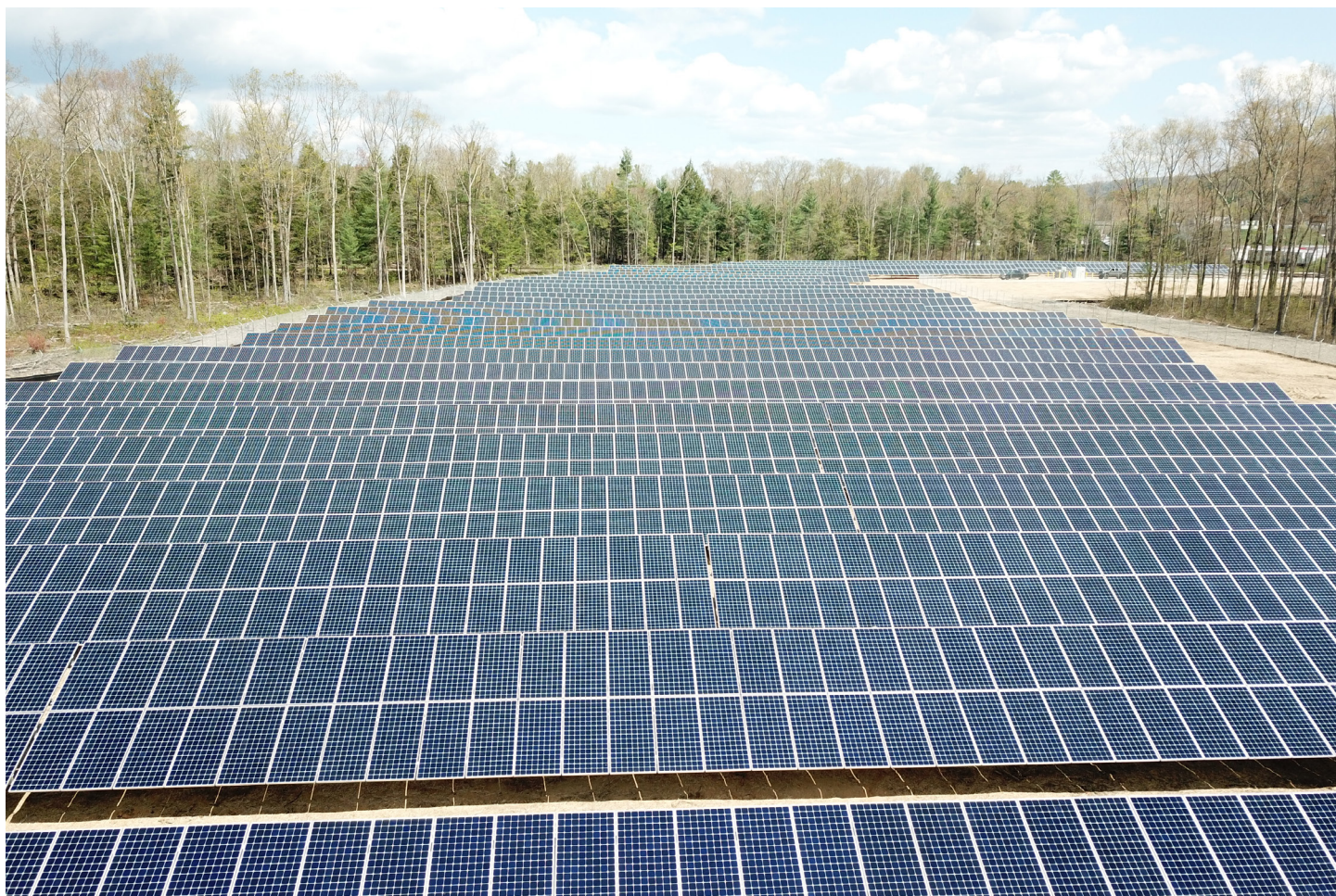
Solar panels installed at Canaan, CT site. A total of 2.9 mega-watts are generated from solar panels at this site.
