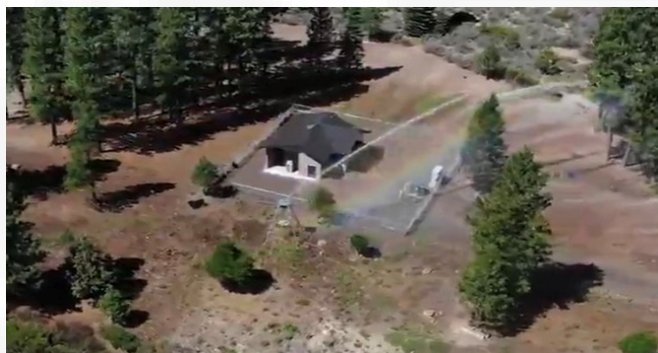
Weed, CA Pumphouse
