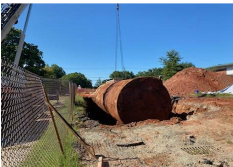
Underground Storage Tank Removal (7/20/2022)
