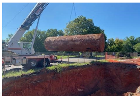
Underground Storage Tank Removal (7/20/2022)
