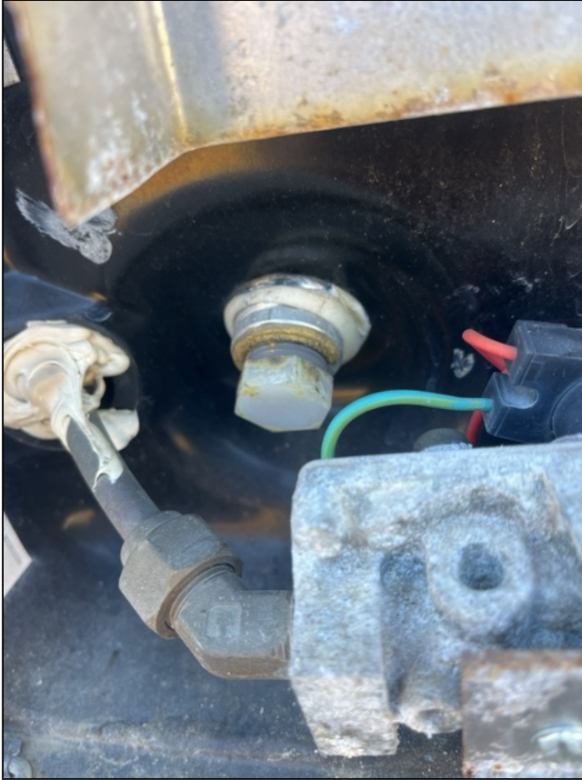
Water heater drain plug
