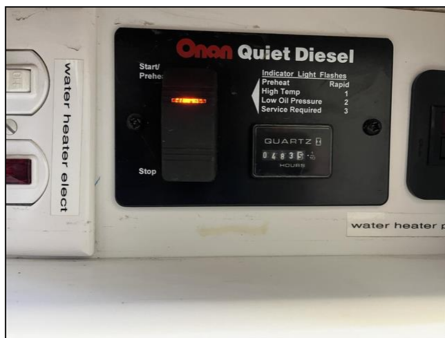
Generator Control Panel
