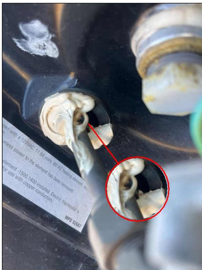
Water heater rubber grommet
