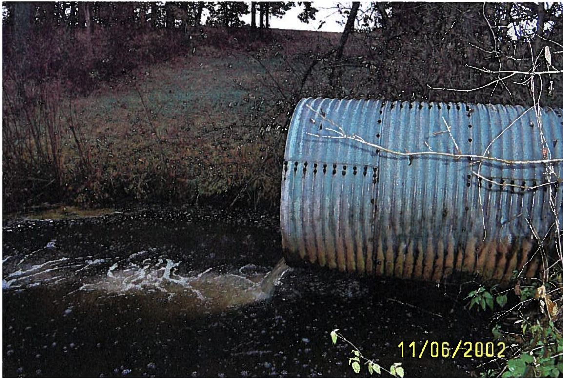
Figure 15. Drop culvert with plunge pool near Ayers Lake
