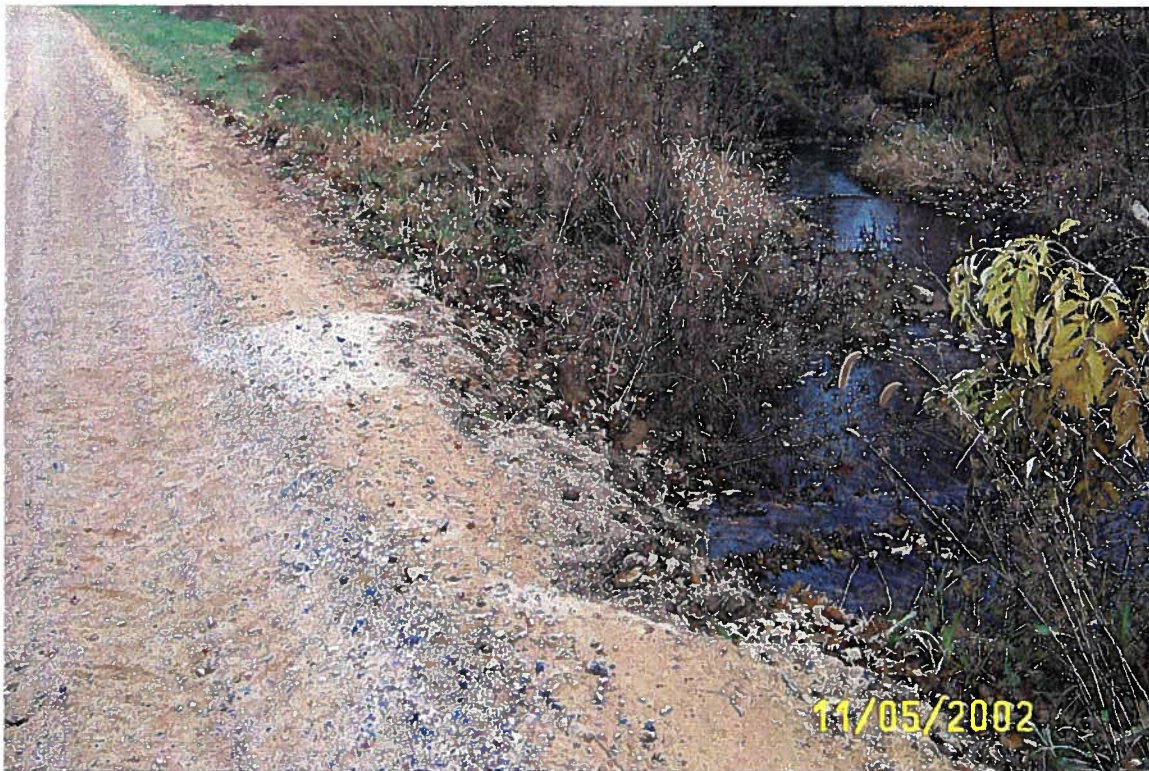
Figure 13. Crossing erosion entering Four County Drain.
