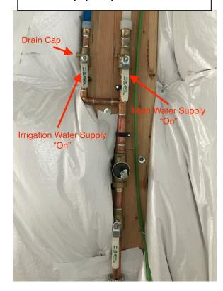
Step 7: After turning on the main irrigation valve, confirm that no water is leaking from the main irrigation valve inside the home or from the backflow and drain cap outside. If leaking, please shutoff main irrigation valve inside the home, and contact Westwind Management Group. Leave the backflow ball valves in the closed position. A GVR Landscape Irrigation technician will open the backflow ball valves to inspect the irrigation system.
