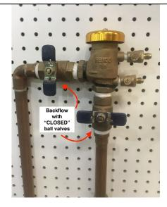
Step 2: Confirm that the drain cap on the elbow below the backflow is closed finger tight (do not over tighten with a tool).
