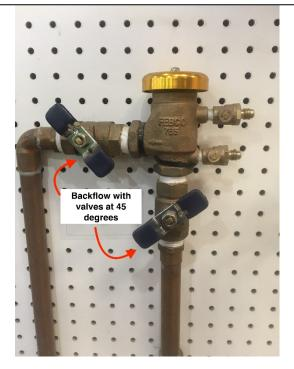
Step 3: Turn both ball valves on the backflow to the "CLOSED" position.
