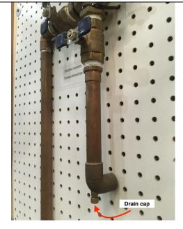
Step 4: Locate the main irrigation shut off valve inside your house (typically located inside a closet in the home).
