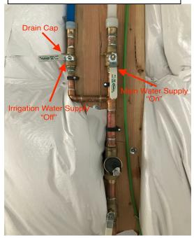
Step 5: Confirm that the drain cap on the main irrigation valve is closed finger tight (do not over tighten with a tool).
