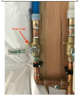
Step 6: Turn the main irrigation valve inside the home to the "ON" position. A rush of water will be heard and should stop quickly.
