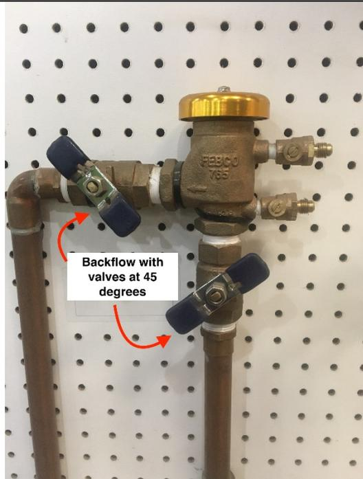
**Step 2: Confirm that the drain cap on the elbow below the backflow is closed finger tight (do not over tighten with a tool).**
