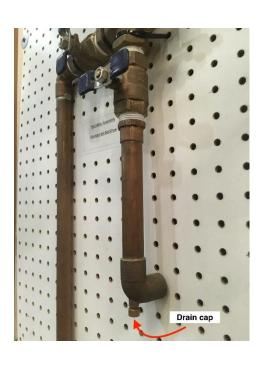
Step 5: Locate drain cap inside home and remove, draining the water. Use a cup or bucket to catch the water
