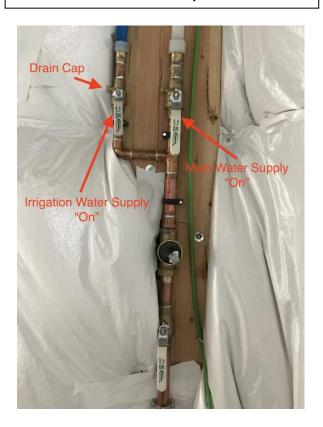
Step 3: Locate the backflow outside of the house. Turn both ball valves on the backflow to the "45" position.
