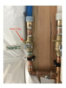
Step 6: Once drained replace the drain cap. Finger tight only.
