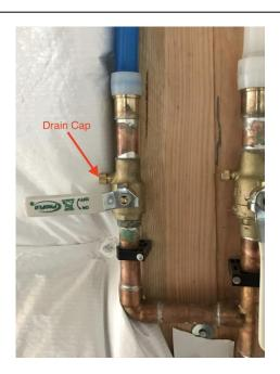
Step 7: After turning off the main irrigation valve, confirm that no water is leaking from the main irrigation valve inside the home or from the drain cap inside. Leave the backflow ball valves in the "45" position. A GVR Landscape Irrigation technician will winterize the backflow, manifold and valves outside the home.
