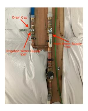
Step 4: Locate the drain cap and untwist till water starts to drip.
