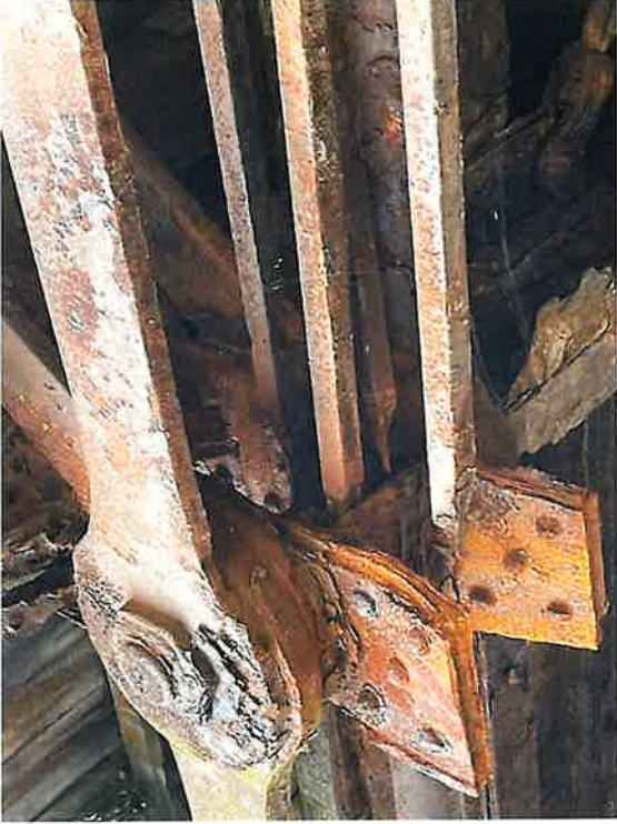
North Truss at L2-L3 (2024) *Continuous deterioration of remaining U-Bar will cause failure of lower Chord L2-L3
