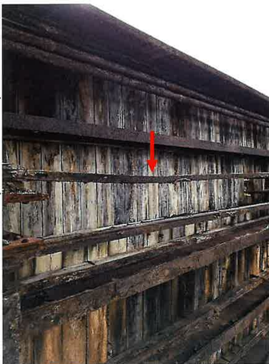
Center South Truss at L1-L2 (2024) *Continuous deterioration of end strut will cause a falling hazard. This end strut is not part of the load path.
