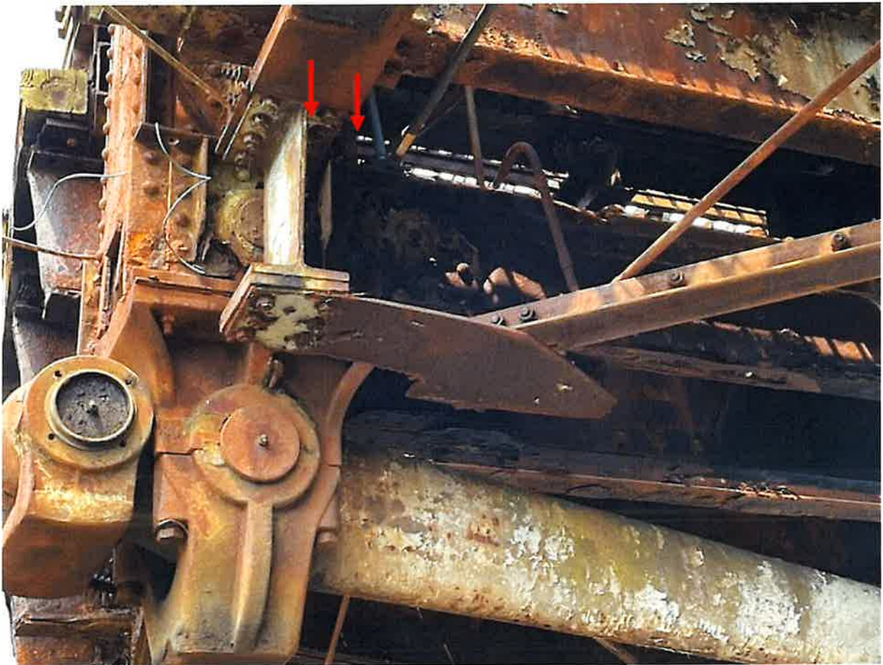
Photo 4. Span Swing, Center North Truss, Lower Chord, L9-L10 (Looking True North) The south channel web and top flange are buckled. Channel webs have up to 1/4" loss. The top and bottom flanges have rust holes
