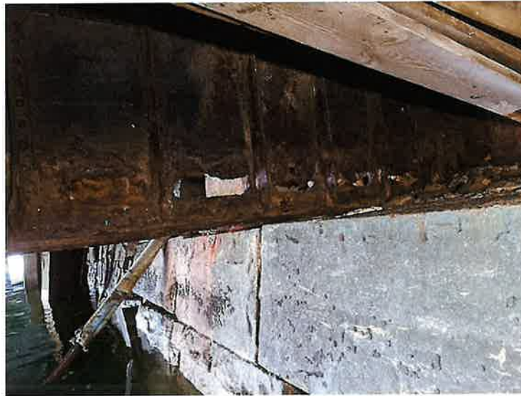
Photo 23: Approach Span 3. Girder P, Between Floorbeams FB5 and FB6 (Looking North) The approach fixed span girders typically have rust holes at the bottom of the webs and severely deteriorated bottom flanges.
