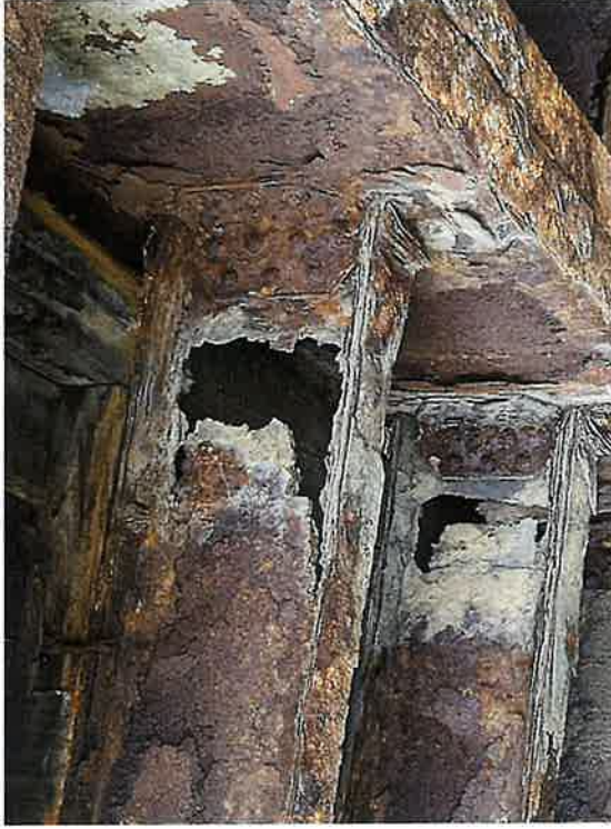
North Bay, Btw FB2 & FB3 – Stringer S4 (2024) *Progressive deterioration of existing rust hole since the 2017 inspection.
