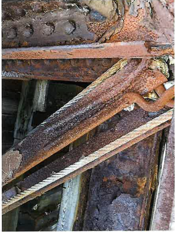
North Truss at L2-L3 (2024) *Continuous deterioration of remaining U-Bar will cause failure of lower Chord L2-L3
