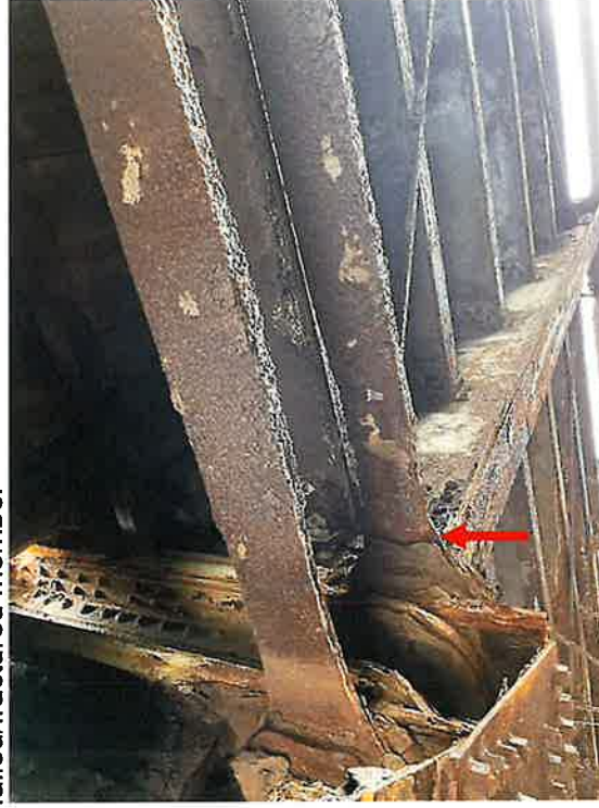
Center North Truss at L26U27 at L26 (2024) *Continuous deterioration of diagonal member will lead to failed/fractured member
