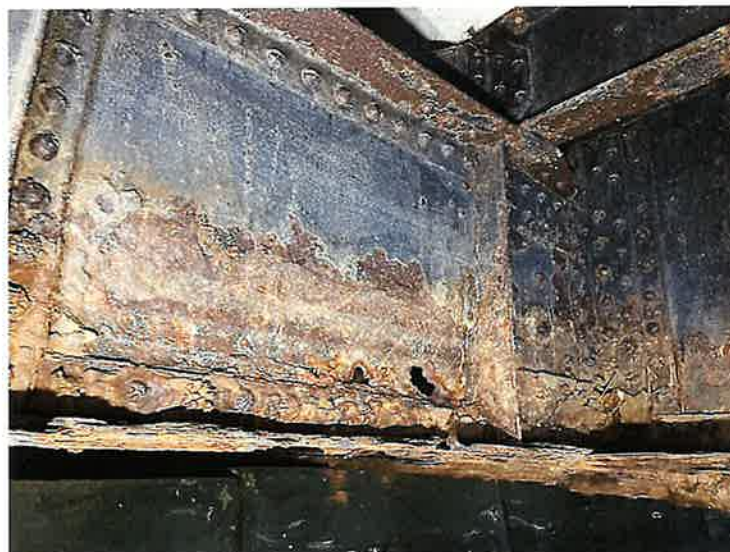
Photo 24: Approach Span 3. Floorbeam FB5, Between Girders GO and GP (Looking East) The approach fixed span interior floorbeams typically have small rust holes and section loss along the bottom of the web
