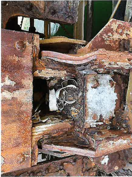
Pier 2, Center South Truss L23 Bearing (2024)
