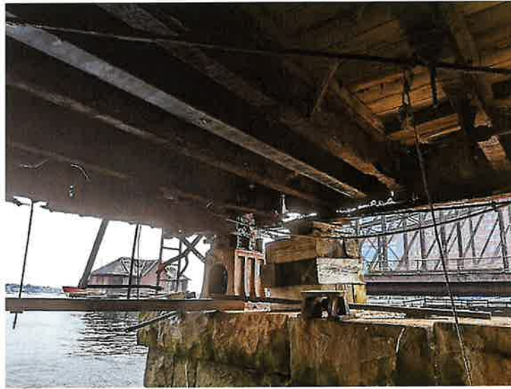
Photo 9: Approach Span 1, Pier 1, North Bearing L8 (Looking Northeast) The pier bearings typically have adjacent timber cribbing.
