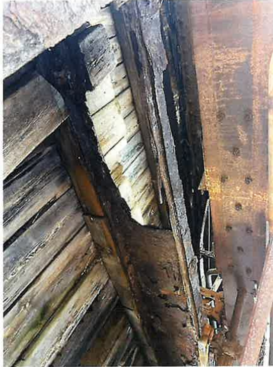
South Bay, Btw FB23 & FB24 – Stringer S1 (2024) *Advanced deterioration of existing rust hole since the 2017 inspection.
