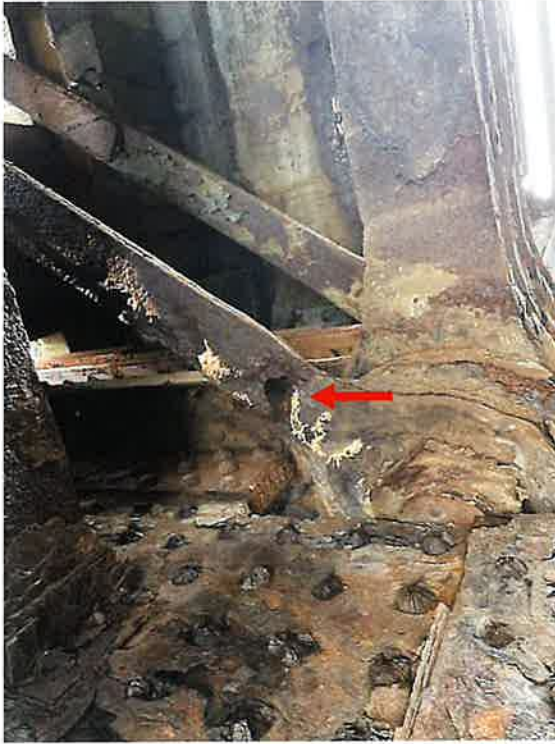
Center North Truss at L26U27 at L26 (2024) *Continuous deterioration of diagonal member will lead to failed/fractured member
