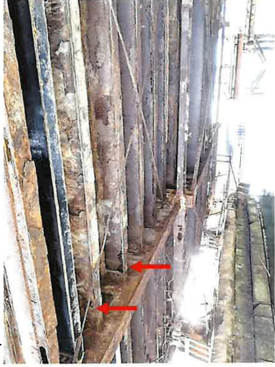
North Bay, Btw FB2 & FB3 – Stringer S4 (2024) *Progressive deterioration of existing rust hole since the 2017 inspection.
