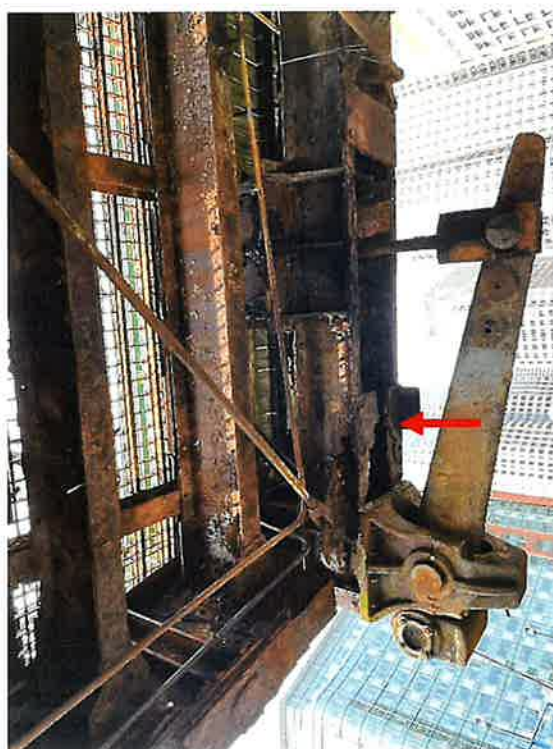
North Truss at L9L10 at L9 (2024) *Advanced deterioration of existing rust hole since the 2017 inspection.
