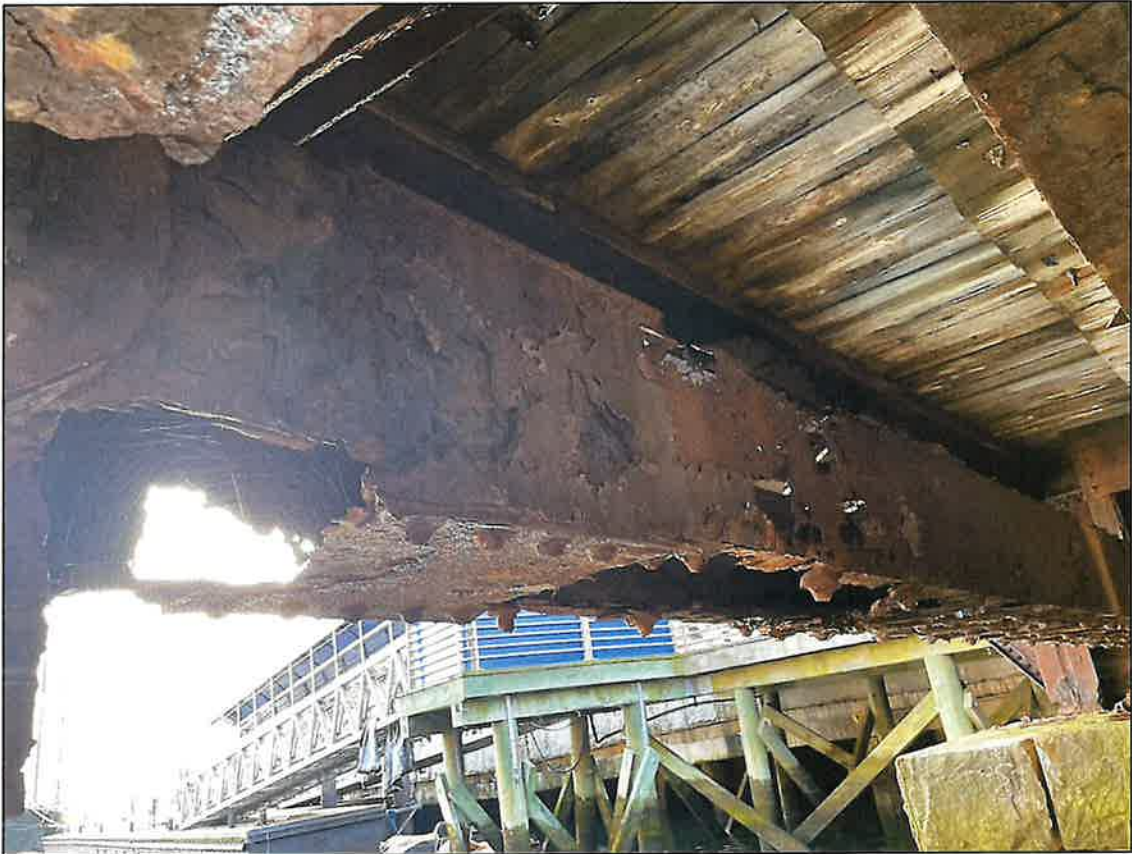
Photograph 6: Detail of stringer deterioration at span 2 (easterly fixed, approach span), and missing mortar from pier 3 looking northeast (August 2024).
