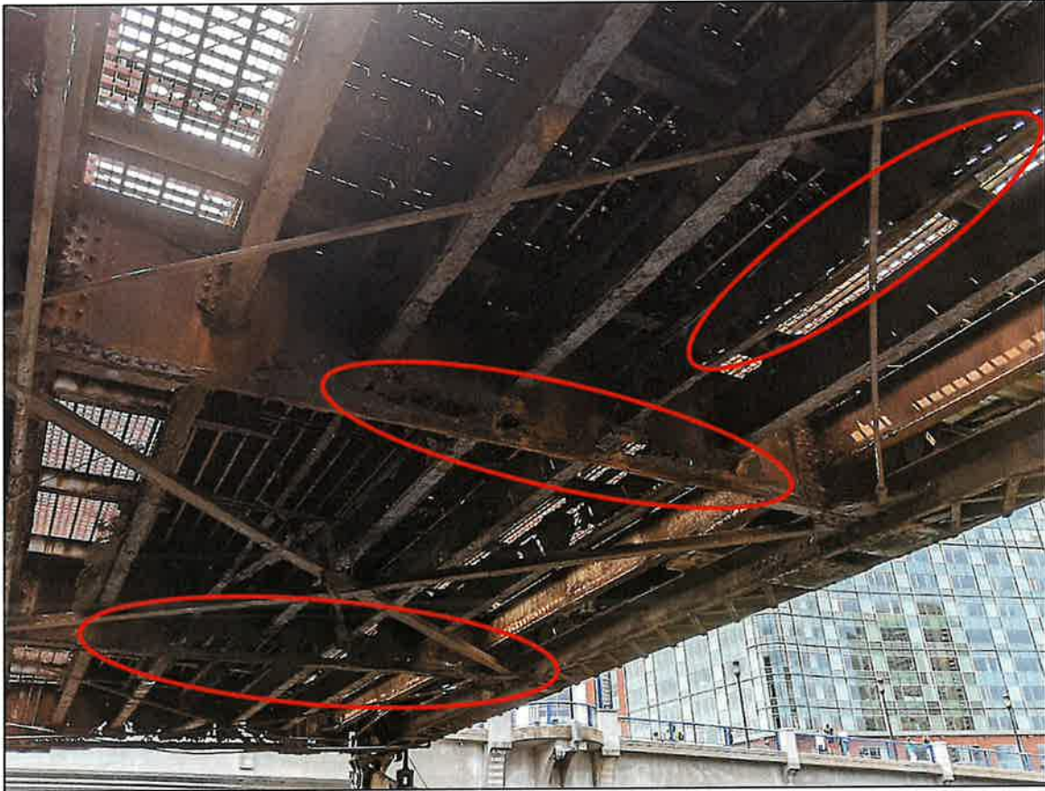
Photograph 5: Section loss at stringers and floor beams of swing span, looking southwest. (August, 2024).
