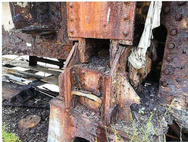
Photo 10: Approach Span 2, Pier 2, Center North Bearing L23 (Looking East) The pier bearings typically advanced deterioration with rust holes and pack rust.
