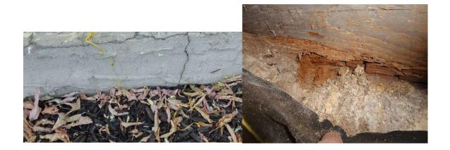
3) Concrete "curb" hiding a wood foundation at the exterior. The foundation appeared to be concrete at first when walking around the exterior.
