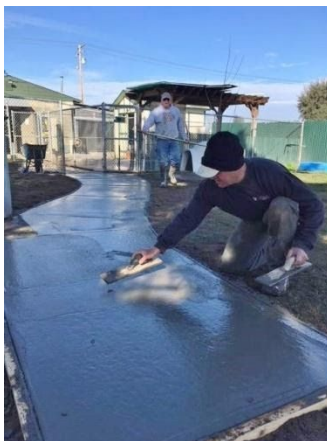
OSPA members construct a new sidewalk in the dog play yard.
