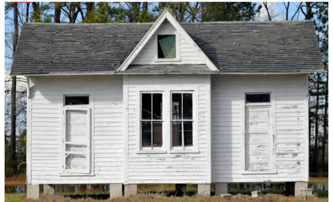
Old Westover Train Station
