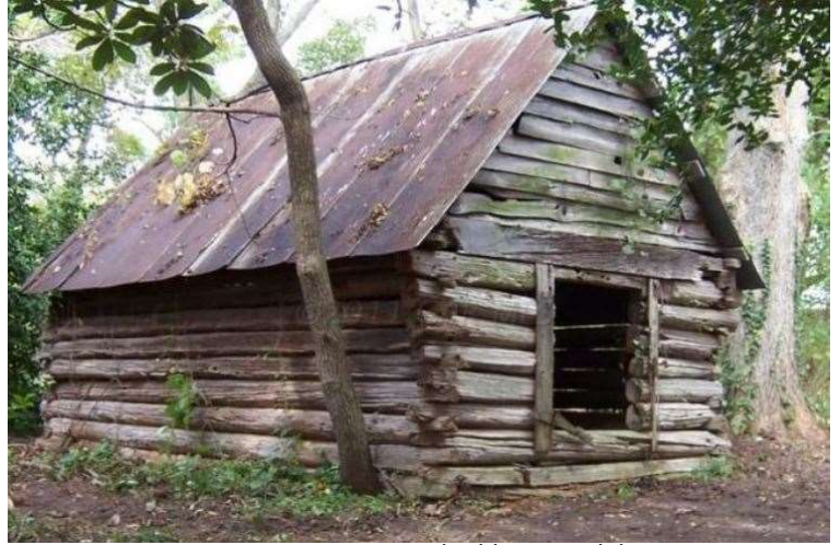
Log outbuilding on Glebe House property (example of period log structure)
