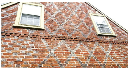
Brick glazed header pattern and dog-tooth bricks, Makepeace
